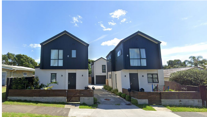
Figure 5: ‘Sentinel’ standalone homes
