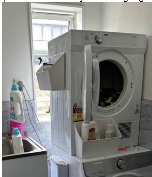
Figure 24: Open window in laundry at back of garage
