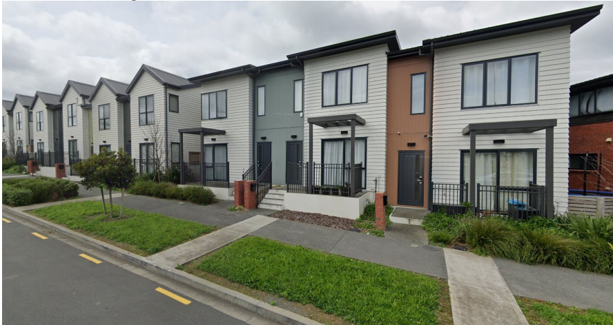
Figure 28: Blinds closed on living room and bedroom windows that overlook the street
