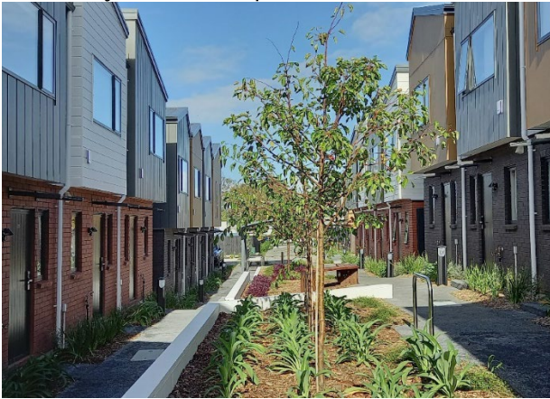
Figure 46: Kitchen windows and glazed front doors overlooking a shared pedestrian accessway, and landscape buffer
