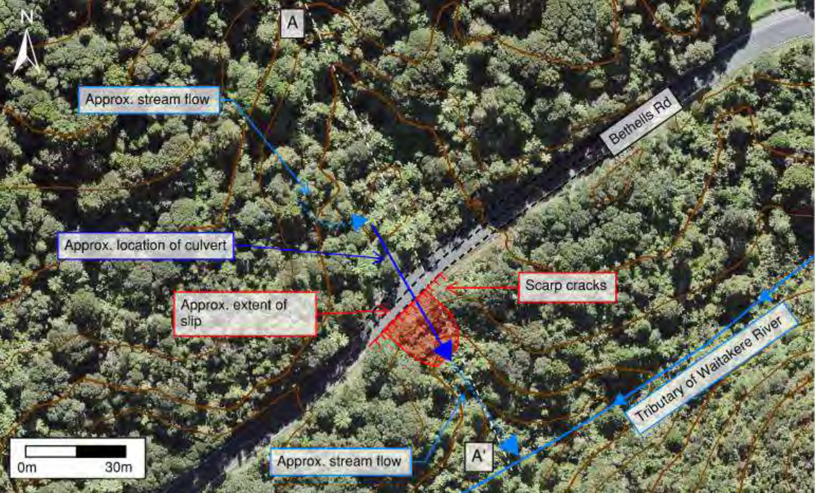
Photo O-11. Bethells Road Slip RP 2.922-2.942, Geotechnical Assessment Report (BECA for Auckland transport)
