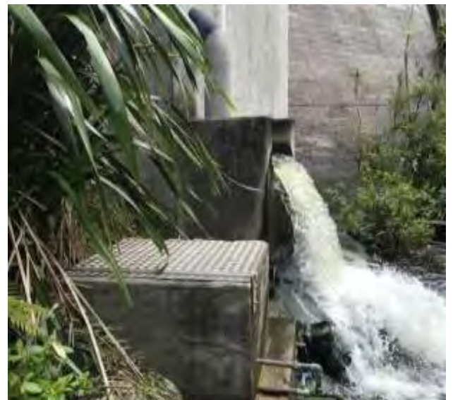
Photo O-16 Waitākere Dam trap / fish path and trap
