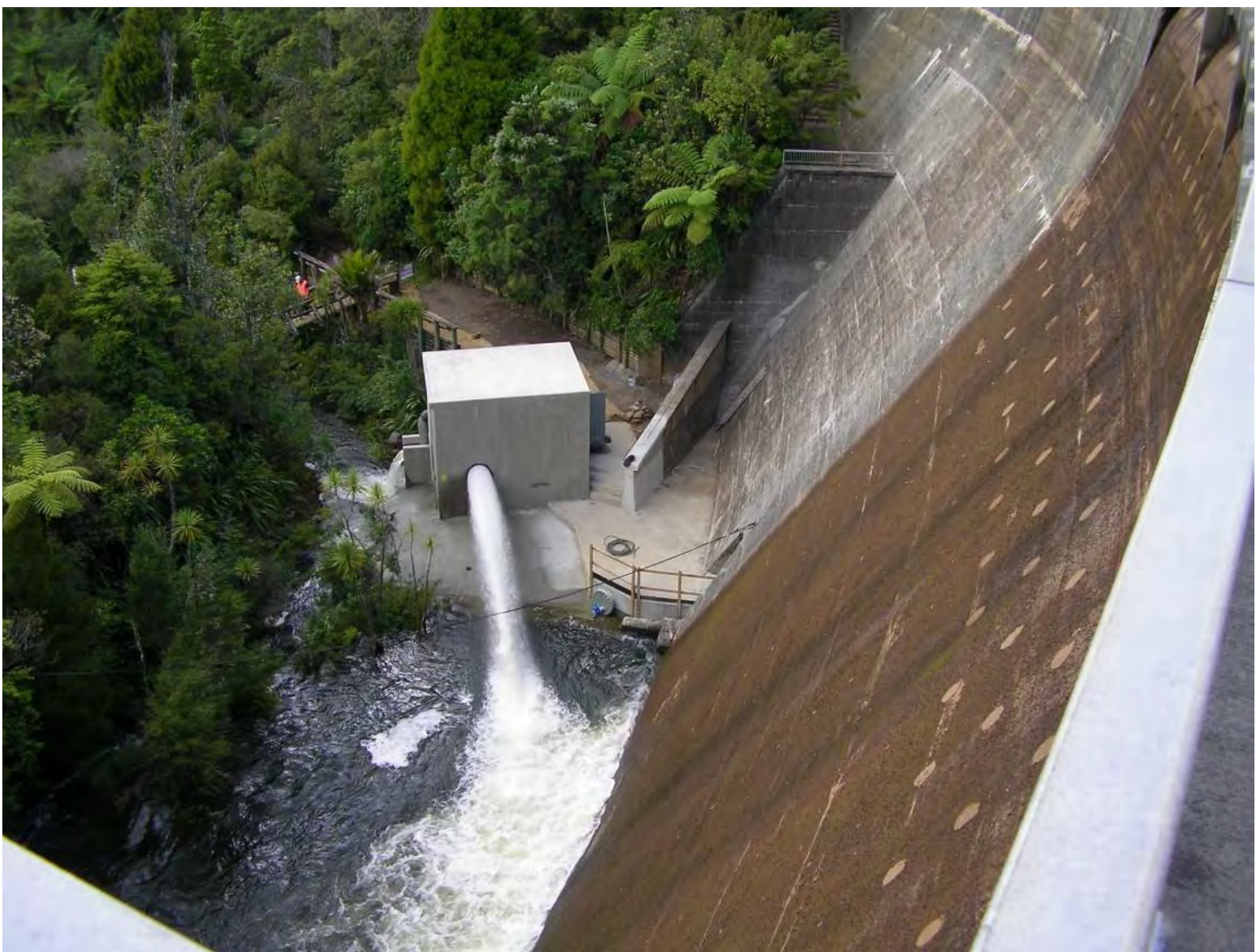
Photo 0-19 Waitākere Reservoir Free Discharge Valve in operation (WSL)
