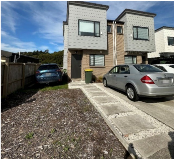
Figure 20: Parking for three cars was created at this duplex by placing bark over the lawn
