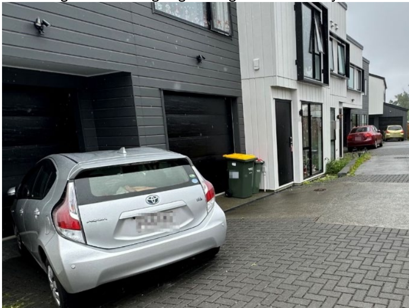
Figure 22: Cars parked at angles in front of garages along shared driveway
