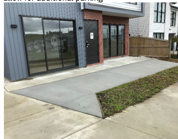
Figure 4: Front yard landscaping and outlook from living areas converted to concrete pad to allow for additional parking
