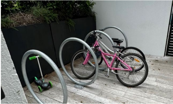
Figure 35: Bikes and scooter stored by Sheffield racks in apartment building
