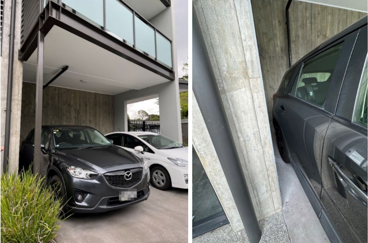
Figure 25: Lack of space to open car door in carpark
