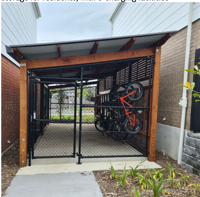
Figure 26: Secure and weatherproof communal bike storage for residents, with e-charging facilities
