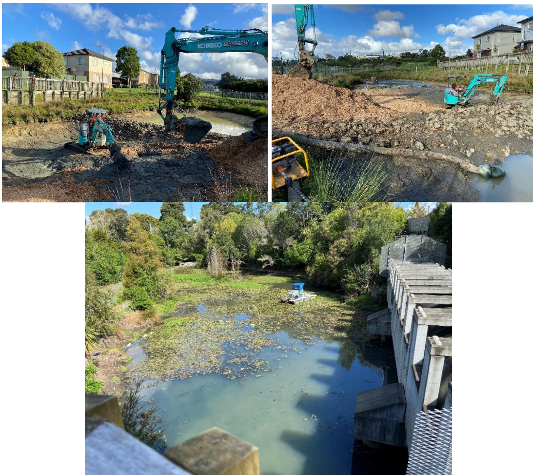
Figure 1. Upper row: digger excavating sediment from Sunnyvale stormwater pond. Lower image: dredge removing sediment from Van Dammes Lagoon.
