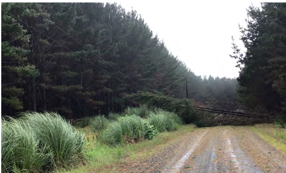
Image: Uprooted trees damaged power utilities in Pouto, Northland. Source: Northpower
