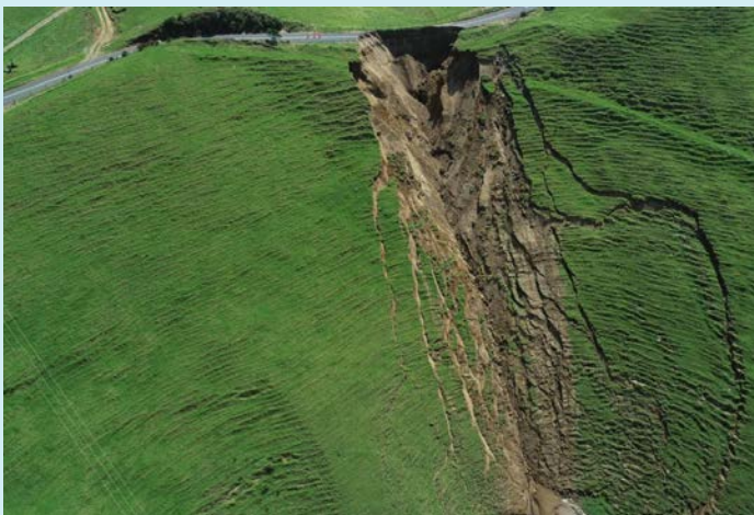
Major slip on a key road in the Āwhitu Peninsula
