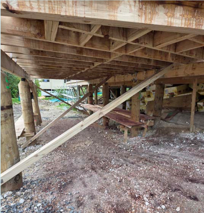
Progress of a house being lifted
