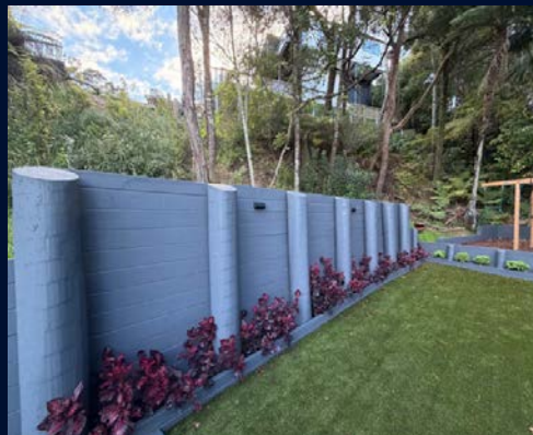
Completed retaining wall to protect the home from future landslips
