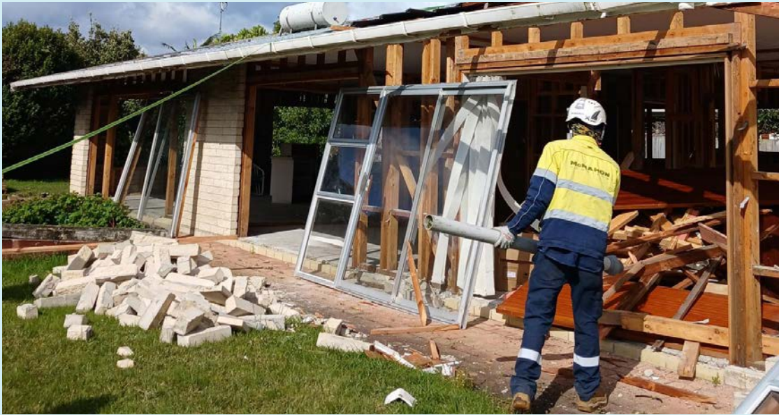
A home being deconstructed in Milford
