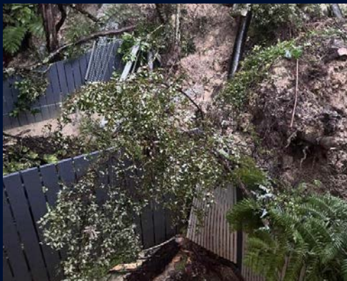
View of the backyard after the landslide from the neighbouring property
