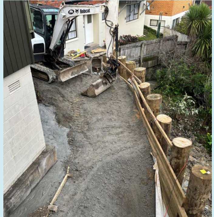
Progress of a retaining wall being built
