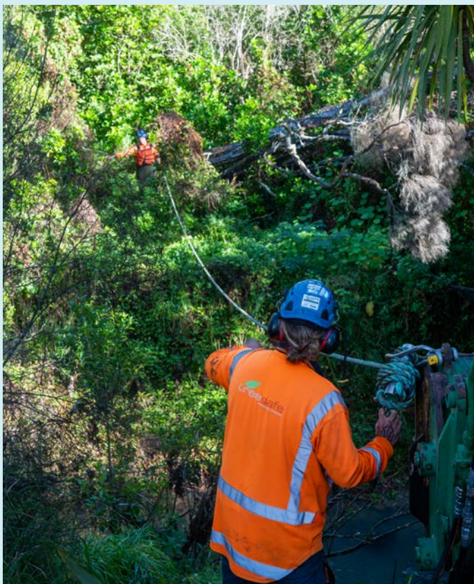
Debris removal at Opanuku Creek in Henderson image by Bryan Lowe
