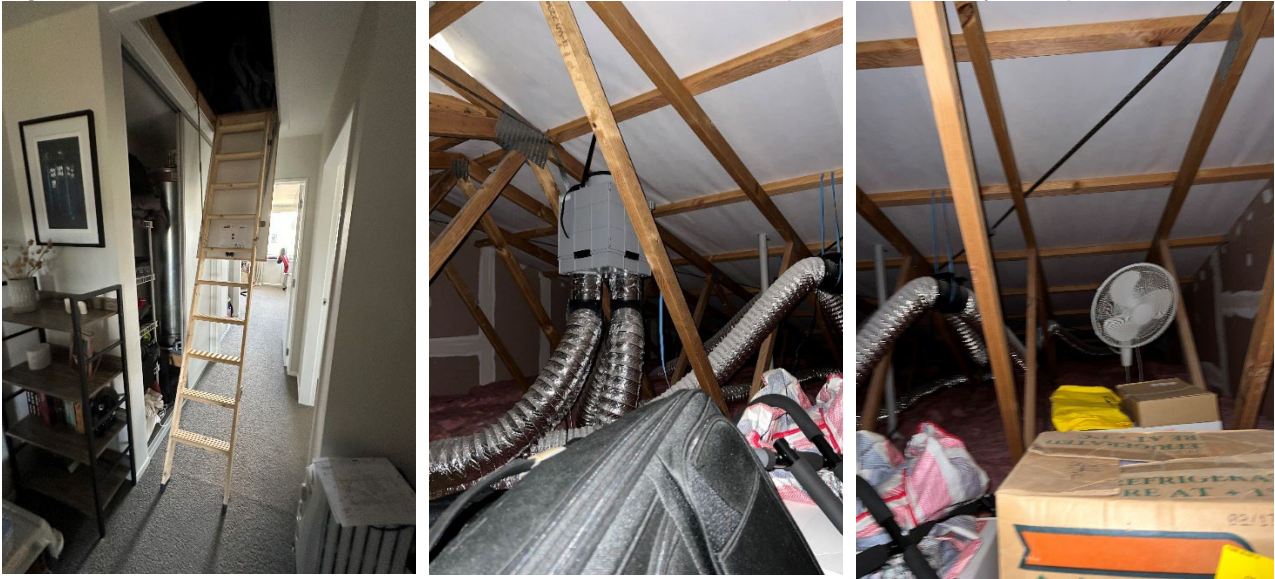
Figure 13: Suitcase and other household items stored in an attic space accessed by a drop-down ladder
