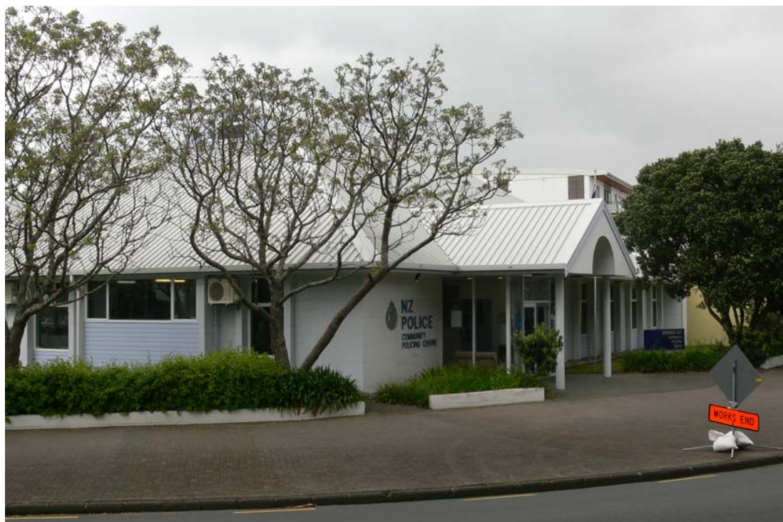
Fig. 13. Brown's Bay Police Station. Photo Archifact.
