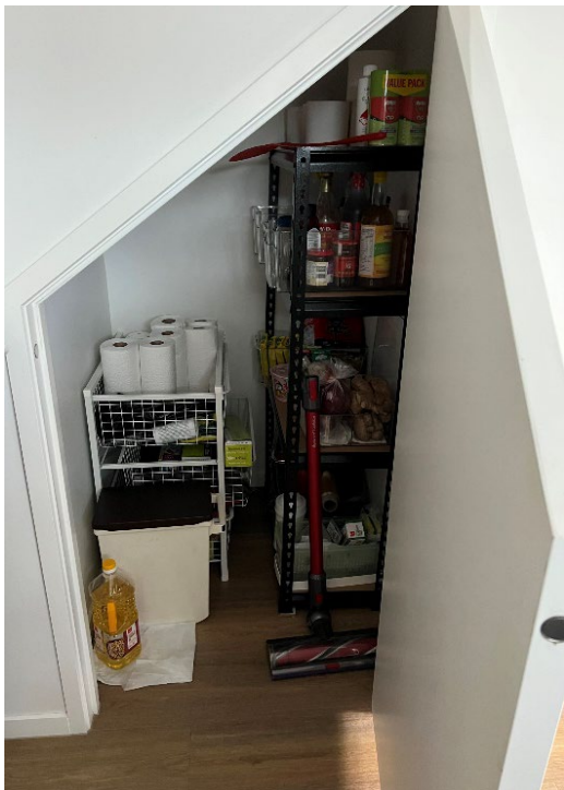
Figure 52: Understairs pantry found to be difficult to access
