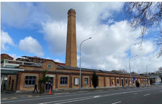
Image: City Destructor Buildings (former), including boiler room, depot perimeter buildings, generator room, battery house, chimney, stables, and destructor building on Victoria Street West, Auckland Central (Category A, ID 02074). It is now used for galleries, workshops, studios, offices, restaurants and retail shops © David Bade (Heritage Unit, Auckland Council, 2024)
