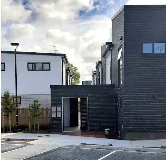
Figure 60: Access control to a rear pedestrian lane serving terraced dwellings
