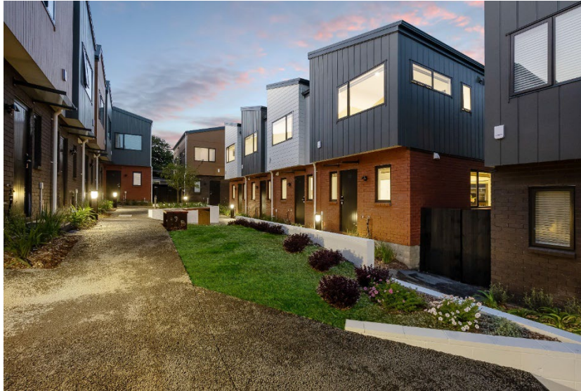
Figure 45: Solar light bollards provided to communal pedestrian accessway
