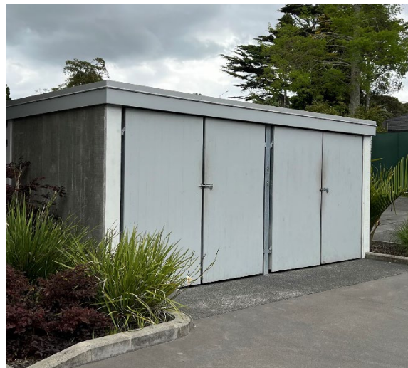
Figure 28: Communal bin storage
