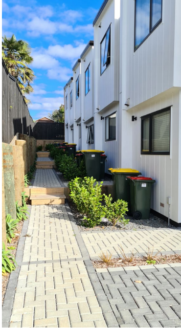
Figure 18: Unscreened individual bins stored outside front door
