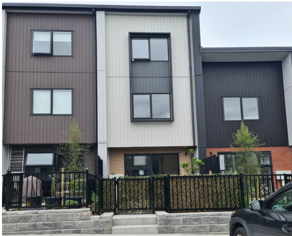
Figure 9: Outdoor living space overlooking a communal parking area, with additional screening added to permeable pool fence
