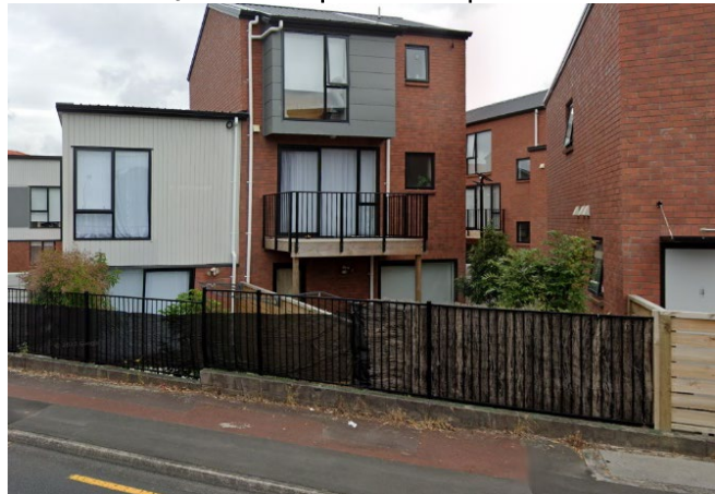
Figure 8: Outdoor living space fronting a street with additional screening (weed mat and brushtix) added to permeable pool fence
