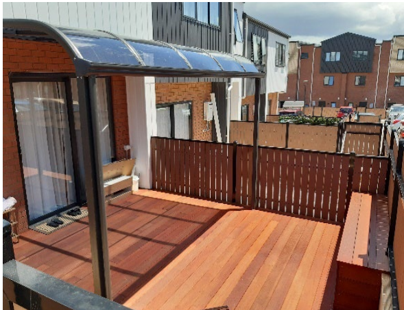
Figure 7: Outdoor living space entirely decked with canopy for shade
