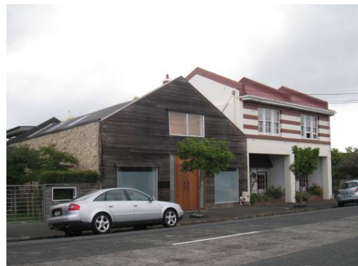
Fig. 37 [right]. 43-45 Queen Street. Photo Matthews & Matthews Architects Ltd, 2010.
