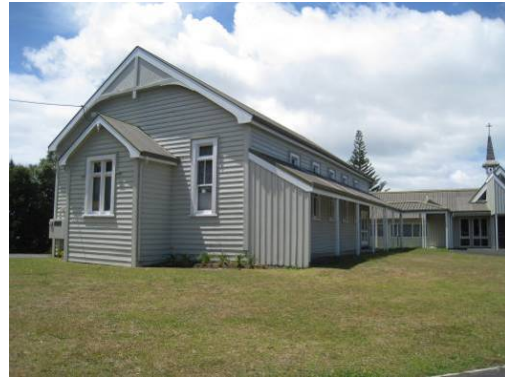
Fig. 56 [right]. The church hall. Photos Matthews & Matthews Architects Ltd, 2010.
