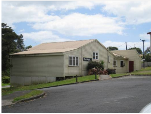
Fig. 71 [left]. Theatre Works, Recreation Drive
