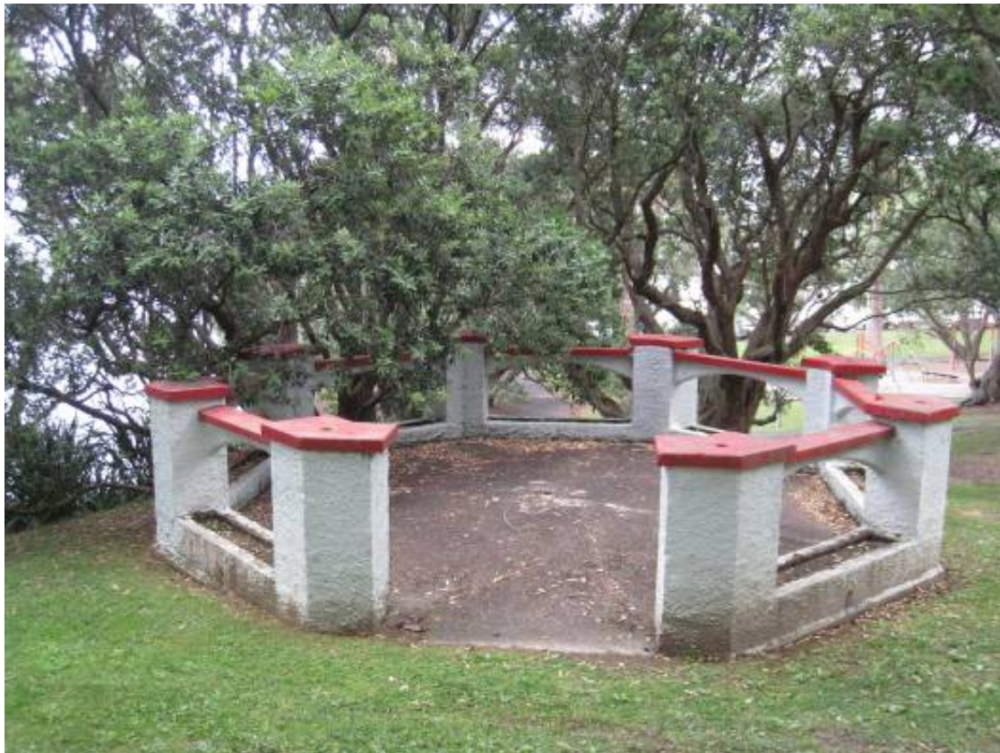
Fig. 30. Base of band rotunda in Hinemoa Park. Photo Matthews & Matthews Architects Ltd 2010.
