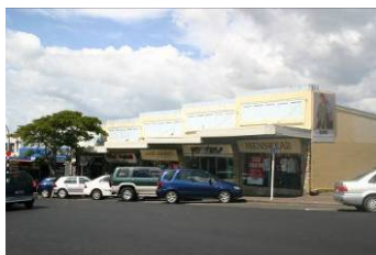
Fig. 22. Highbury Buildings, 14-20 Mokoia Road, built in 1934
