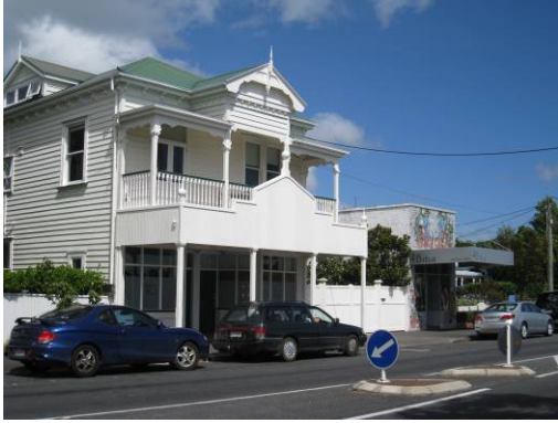
Fig. 47. 144a-146 Hinemoa Street. Photo Matthews and Matthews Architects Ltd, 2010.
