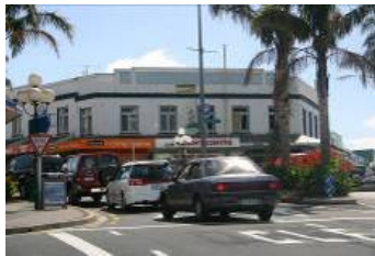
Fig. 20. Payne's Building at 1-5 Mokoia Road built in 1928 54
