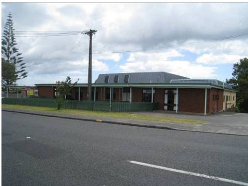
Fig. 27. Birkenhead Baptist Church 25 Birkdale Road. Photo Matthews and Matthews Architects Ltd, 2010.
