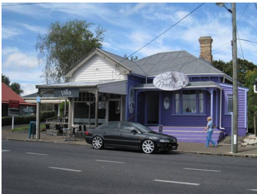
Fig. 50. 134 Hinemoa Street. Photo Matthews and Matthews Architects Ltd 2010.
