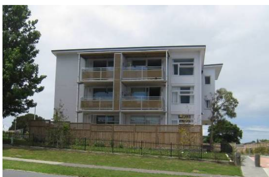
Fig. 21 [left]. 'Star-block' state houses in Lake Road.
