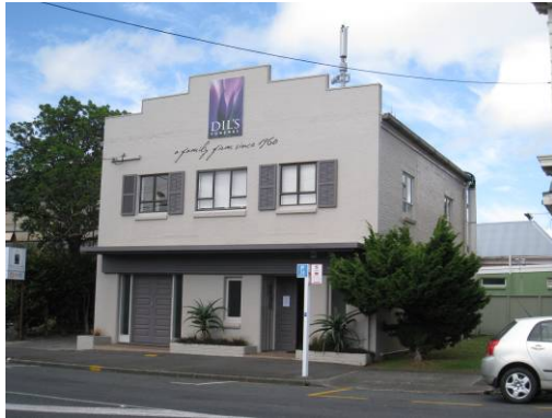
Fig. 55. 92-94 Hinemoa Street. Dills Funeral Parlour. Photo Matthews and Matthews Architects Ltd, 2010.
