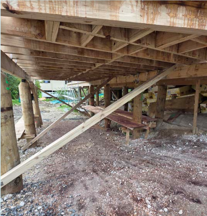
Progress of a house being lifted
