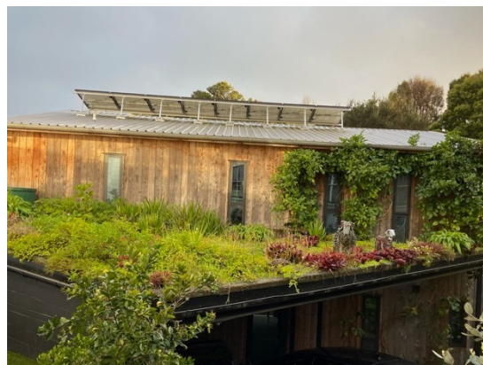
Green roof, rain tank and solar panels at Wiles Ave, Remuera (photo courtesy of Robyn Simcock)
