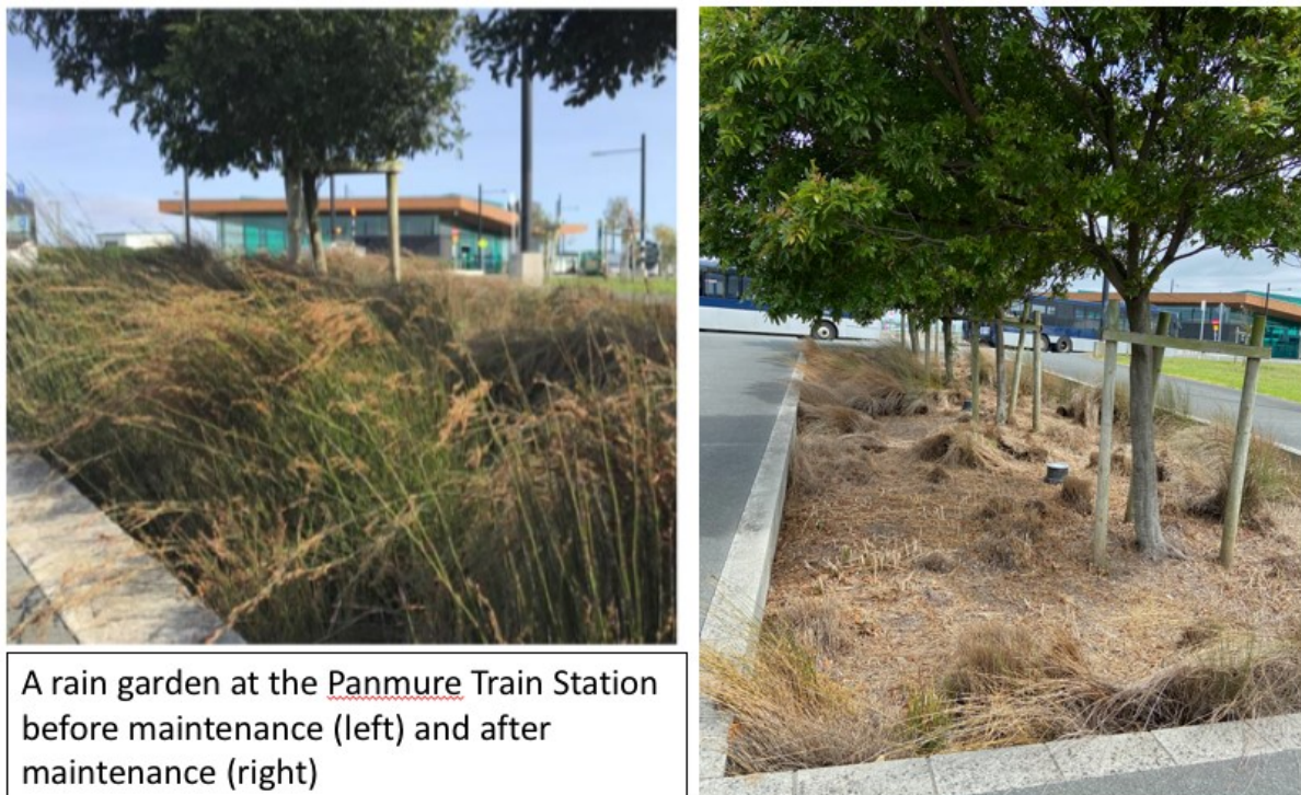
Figure 21 An example of the type of maintenance which is occurring on many rain gardens in Auckland
