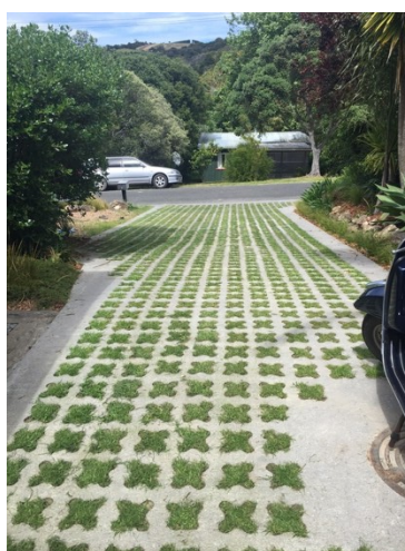
Permeable paved driveway on Waiheke Island (Photo courtesy of Wynand du Toit, Stormwater360)
