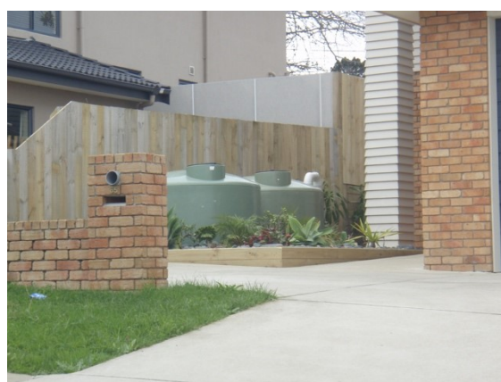
Rain tanks in Rising Way, North Shore
