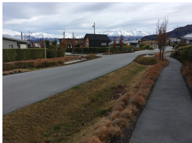
Figure 10 Kirimoko Park, Wanaka: WSD pipeless subdivision with narrow road widths, swales, rain gardens, rain tanks and infiltration basins
