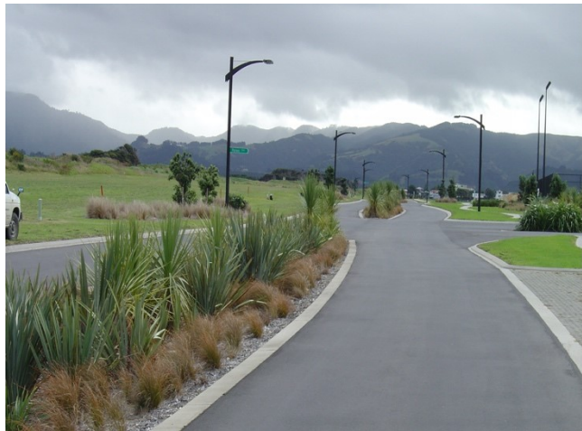
Figure 9 Rain gardens and paving providing water quality treatment and infiltration in Omaha
