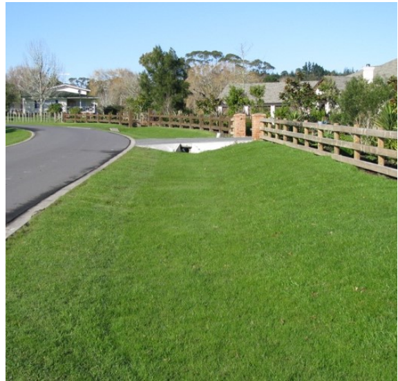
Figure 7 Roadside swales and narrow road widths, no footpaths (Goodland Estates)
