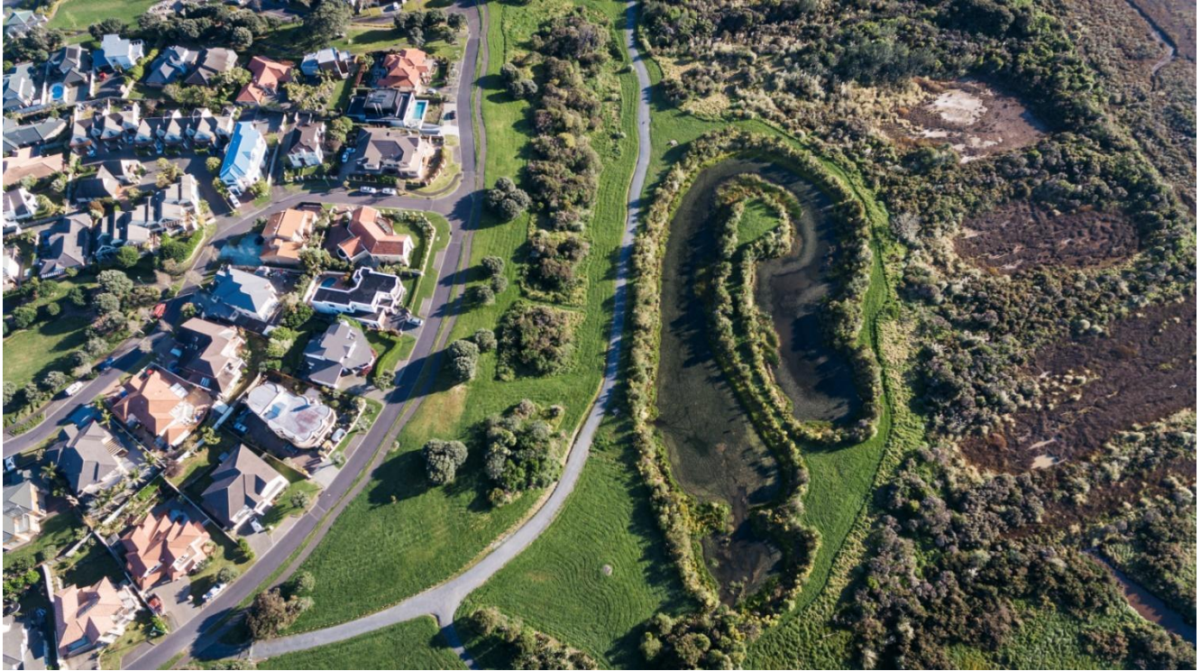
Photo 5: An aerial view of Danica Esplanade Pond, showing the scattered slope planting (between the path and the road) and extensive areas of salt marsh to the east (right of photo). Photo supplied by Auckland Council (2018).
