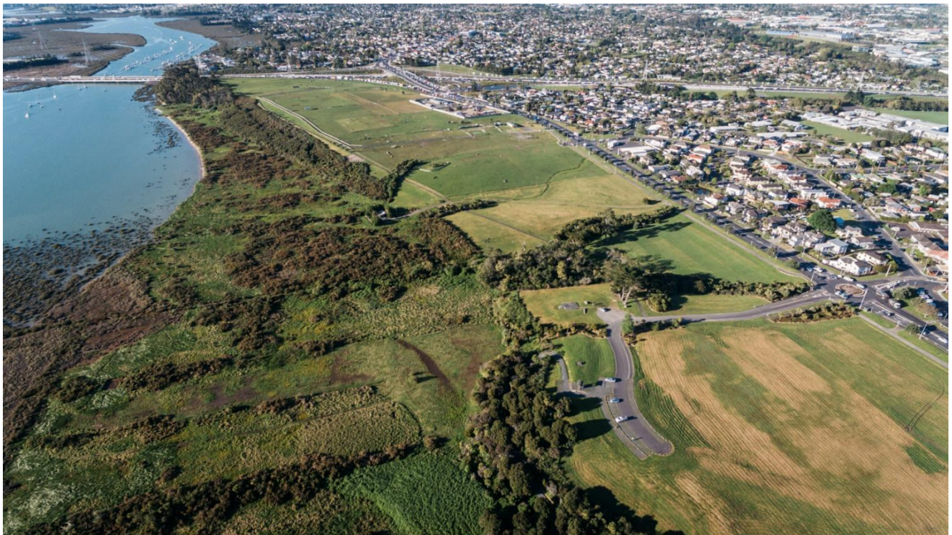
Photo 7: A 2017 drone photo of the central and southern zones, looking south, (photo supplied by Auckland Council).
