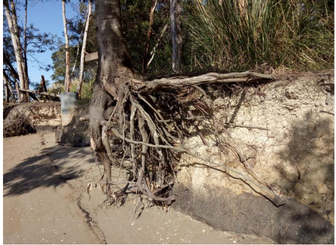
Photo 13: Erosion at the brickworks site. Planting is unlikely to slow erosion as wind-driven waves can undermine the root plate.
