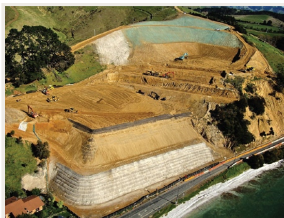
FIGURE 2 Aerial view of the earthworks being undertaken in May 2009 to stabilise the Turei Hill landslides. (Source: Manukau City Council).
