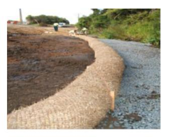
Figure 89: Silt sock used to provide control during final landscaping
