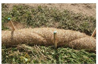
Figure 93: Straw sock secured in place using stakes and bale twine; note the stakes are placed every 600 mm
