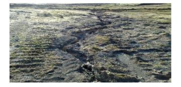
Figure 46: Loss of topsoil and grass seed after heavy rain event. Will require stabilisation and reapplication
