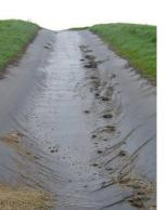
Figure 30: Geotextile lined flume
