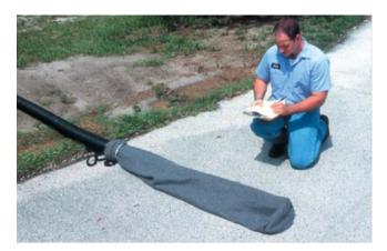
Figure 105: Dewatering bag and pipe sock
