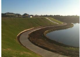
Figure 42: Grass stabilised earthworks site. Batter and building platforms
