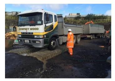
Figure 36: Example of truck wash and shaker ramp
