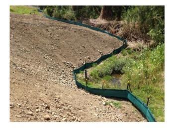
Figure 84: Contours create the same effect as returns in this case
