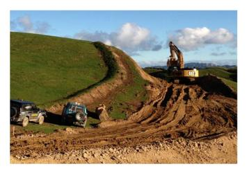
Figure 14: Clean water diversion used to isolate upper clean water flows from the works area
