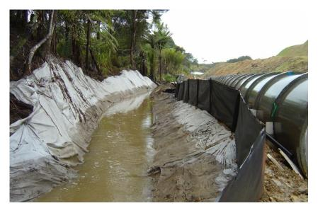
Figure 111: Temporary stream diversion to allow for the installation of a new culvert
