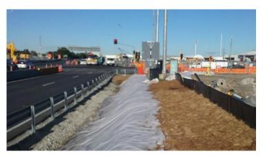
Figure 108: Progressive stabilisation in limited space
