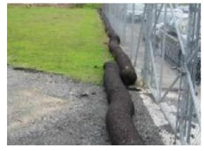
Figure 91: Silt sock with 1 m overlapping joint
