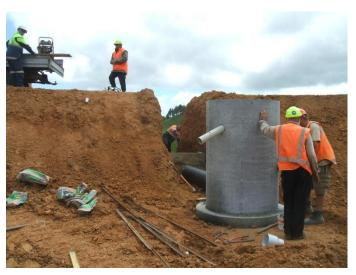
Figure 74: Installation of the outlet pipe and the anti-seep collars
