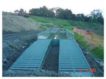
Figure 37: Example of a shaker ramp
