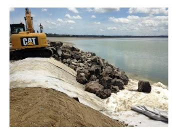
Figure 133: Use of geotextiles and coastal protection rock (Source: SouthernSkies)
