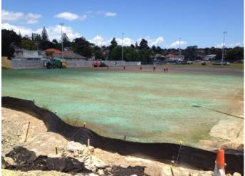
Figure 48: Sports field being hydroseeded. Sediment control remains installed until an 80% grass strike has established
