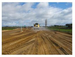
Figure 128: Water truck dampening down the works area
