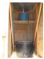
Figure 102: Header tank
