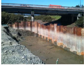
Figure 131: Sheet pile coffer dam (Source: SouthernSkies)
