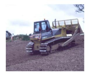
Figure 38: Surface roughening with bulldozer
