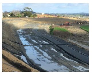
Figure 33: Pipe-drop structures conveying upper water down an exposed slope
