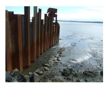
Figure 132: Water draining from a sheet pile coffer dam (Source: SouthernSkies)
