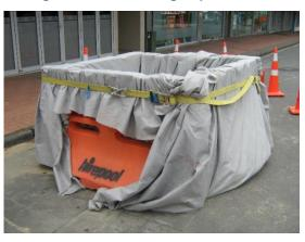
Figure 106: Example of a mobile 'turkeys nest' used for dewatering
