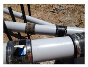
Figure 76: Steel strapping used to attach decant system to horizontal pipework
