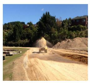
Figure 125: Dust suppression using a water cart
