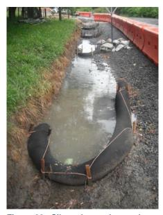
Figure 26: Silt socks can be used as a check structure on a low gradient channel
