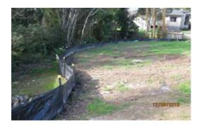
Figure 107: Silt fence
