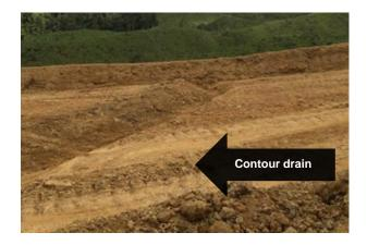
Figure 21: Contour drain
