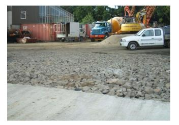
Figure 34: Stabilised entranceway
