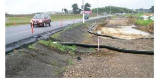
Figure 29: Flume conveying clean water over the works area
