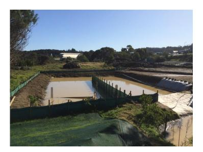
Figure 67: Example of baffles
