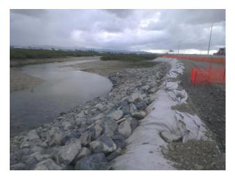
Figure 130: Examples of geotextile filter layer beneath a rock revetment and use of rip rap (Source: SouthernSkies)
