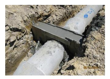
Figure 70: Example of an anti-seep collar
