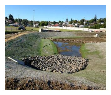
Figure 49: Recently applied hydroseed on a stormwater wetland
