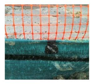
Figure 85: Use of silt fence clips
