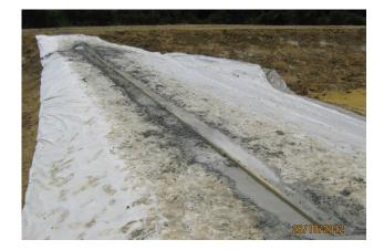
Figure 68: Example of a level spreader
