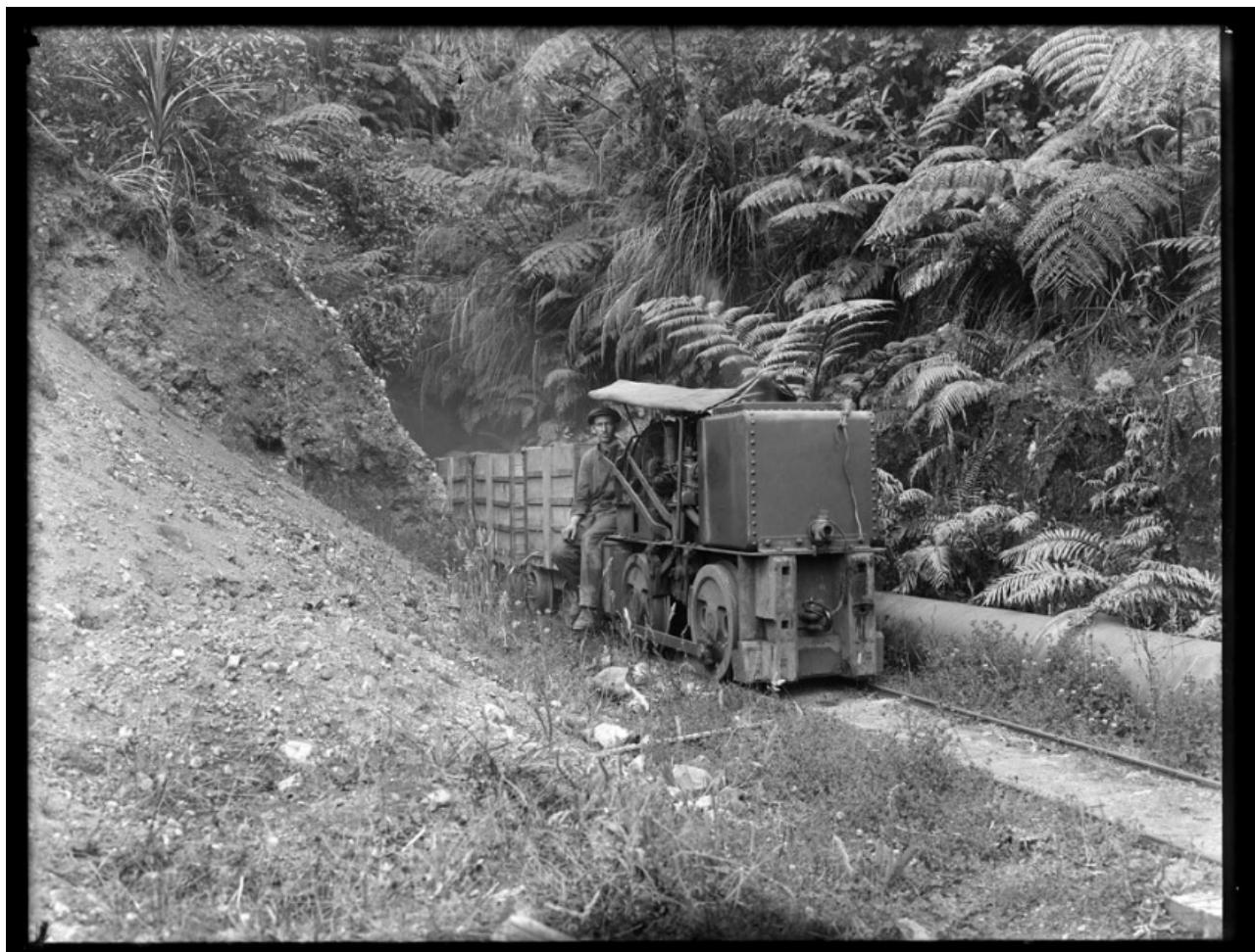
Nihotupu tramline and pipe route during construction of the Upper Nihotupu Dam, with locomotive used to haul construction material to the dam site (Source: Sir George Grey Special Collections, Auckland Libraries, 1-W1784).
