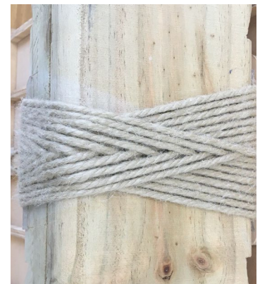
Haumi balustrade binding prototype (Tessa Harris)
