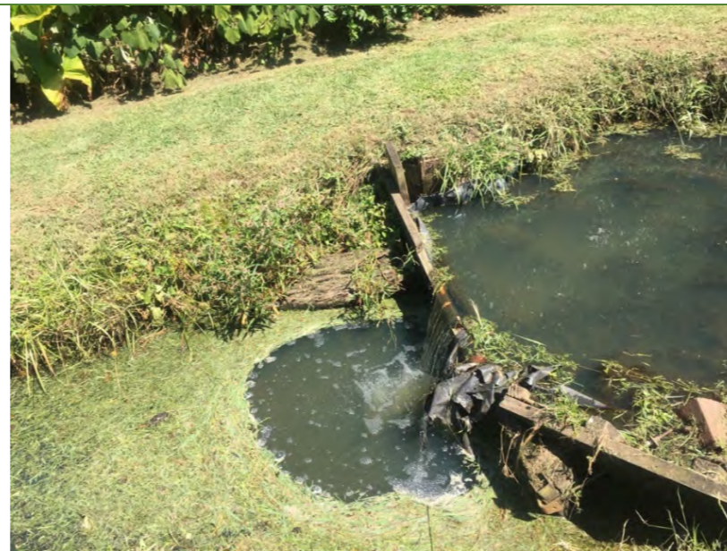
Multiple ad-hoc weirs and dams structures used to create ponding sections of stream.
