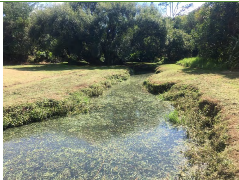
Open channel with dominated by lawn grasses providing limited filtering ability and no riparian shading (Trib ID: GLE_MAIN_3).
