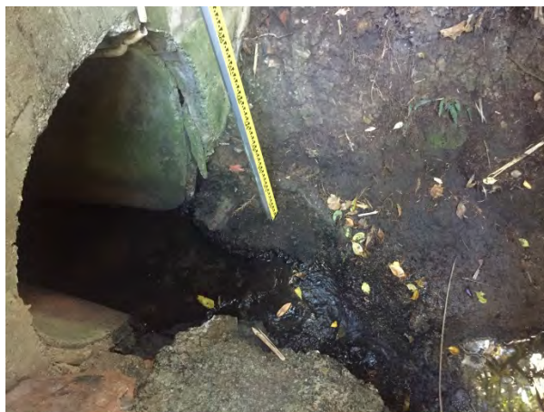
Informal cast in-situ concrete headwall that is cracked and erosion of the bare earth banks on both banks at 53 Clarendon Rd (2000677856).
