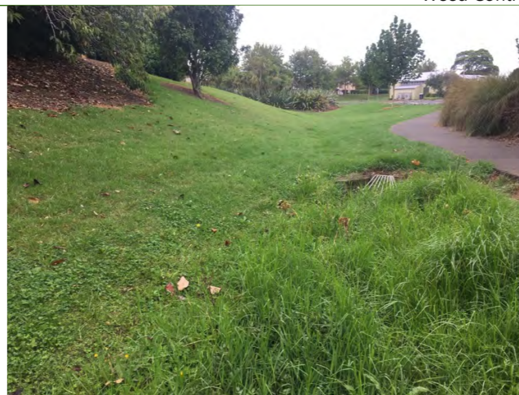
The concrete footpath on TLB of the proposed daylighting site.
