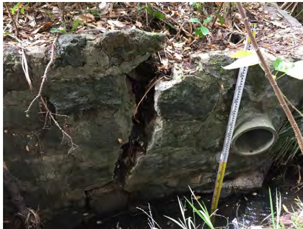
Detached headwall in Dingle Dell Reserve (2000649833).
