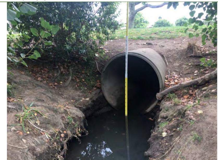
Asset ID 2000229311 with an unconstrained drop height of 1.6m close to the walking path.
