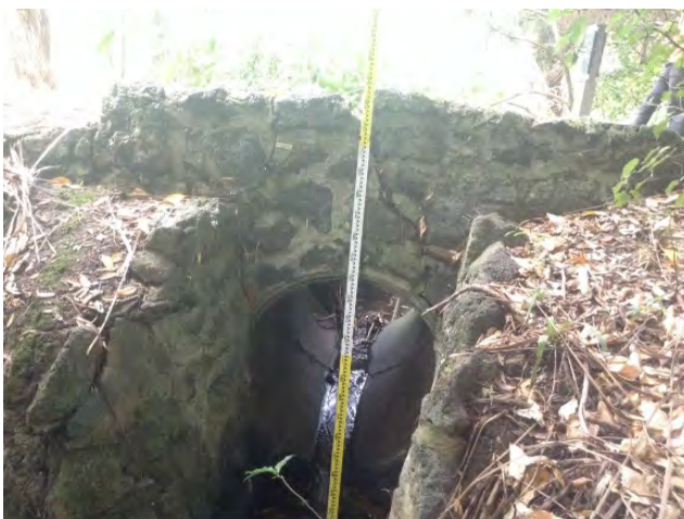
Cracked culvert bridge in Dingle Dell Reserve (EBS_004, EBS_005, EBSP_003).
