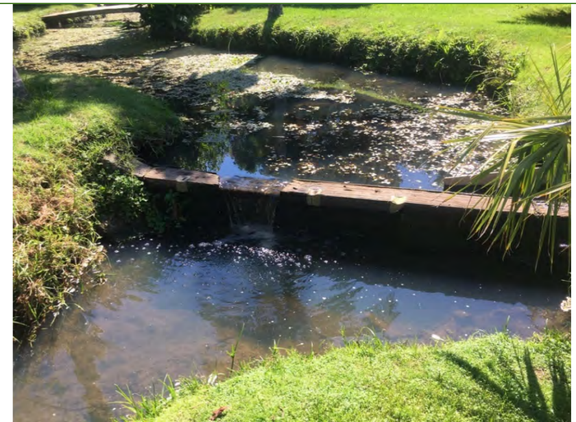
Weirs are complete fish passage barriers (GLE_MAIN_4).
