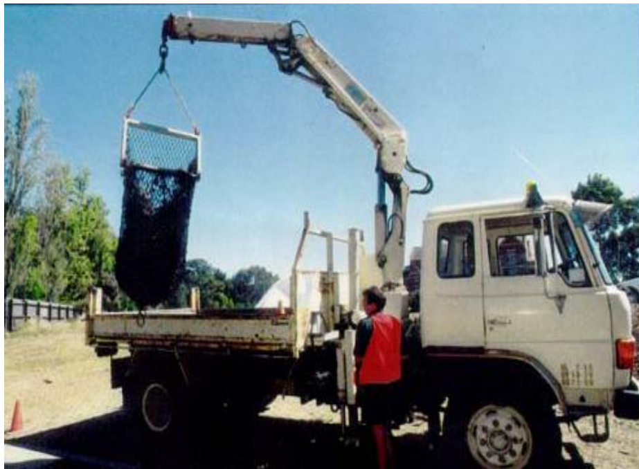
Photo 1: Maintenance of a litter and sediment trap by vacuum (Department of Water 2006)
