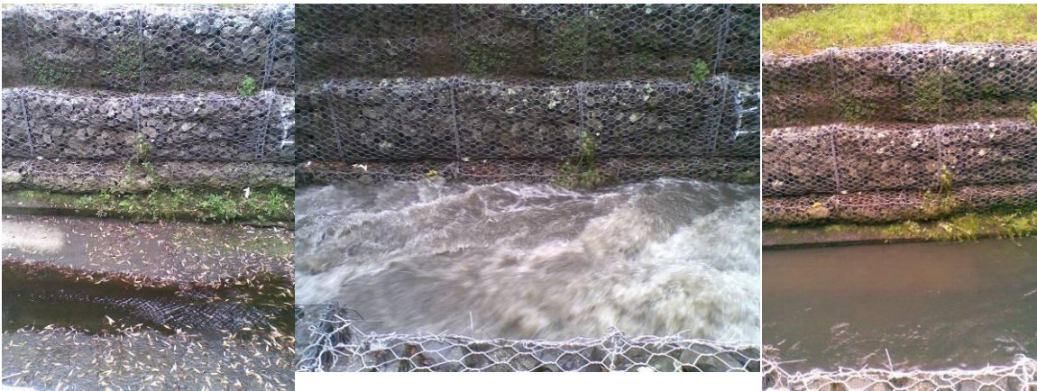
Figure 4: DSAAG site before, during and after the rain event.
