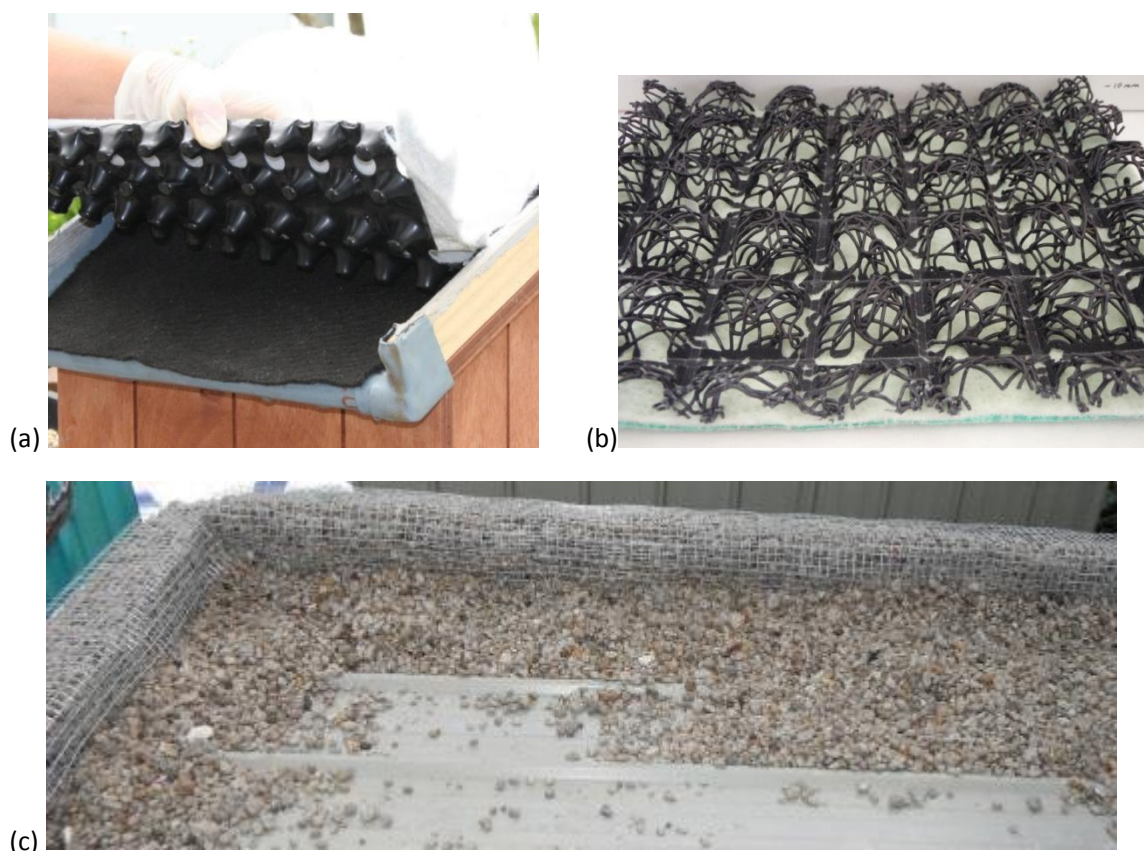
Figure 11. Drainage layers: (a) synthetic “egg-crate” style moulded plastic with “cups up”; (b) plastic mesh; (c) installation of granular drainage layer and edging made from pumice.
