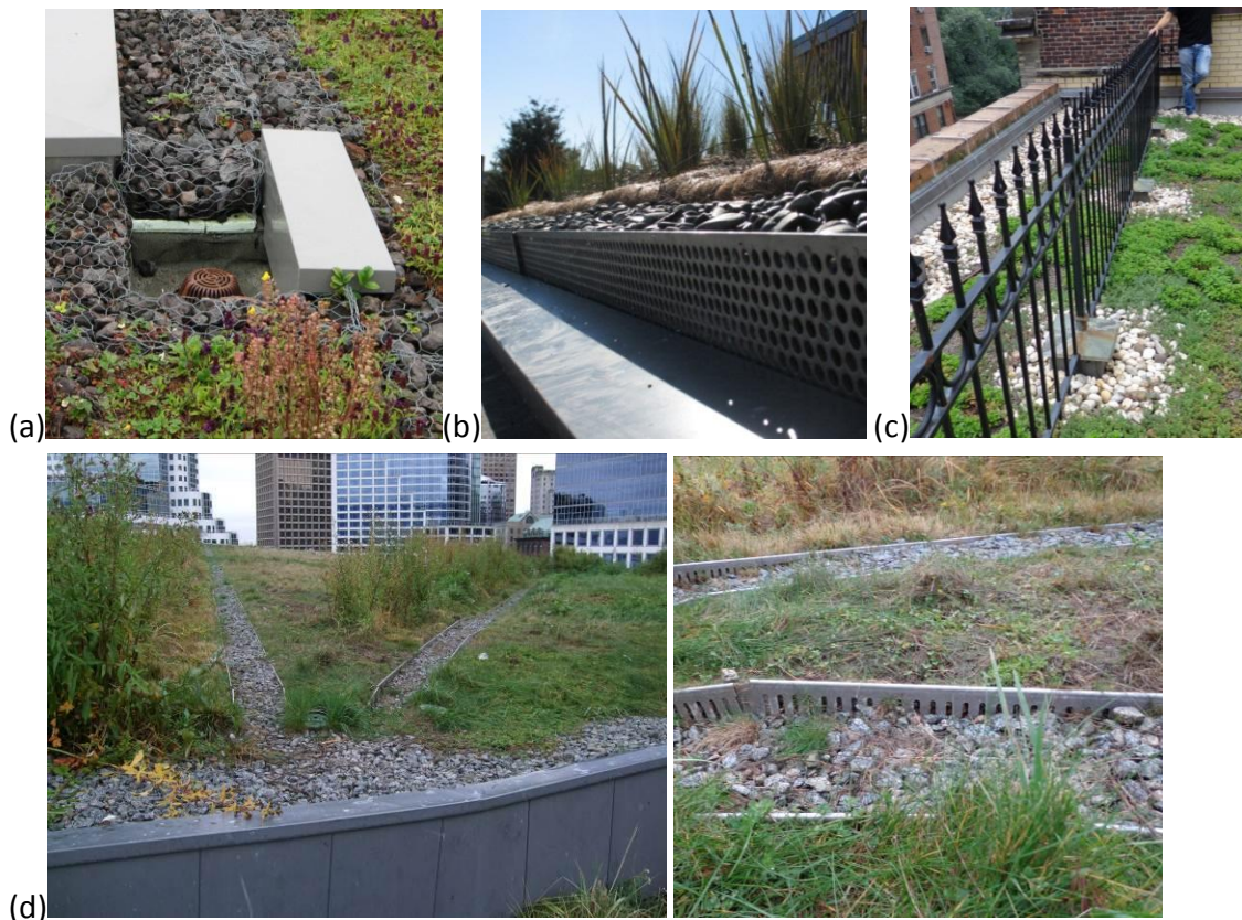
Figure 10. Importance of edging material; (a) scupper inlet and protrusion protection; (b) edging material to promote drainage; (c) protection of footings, cue for building edge; (d) edging material used as a drainage “break” for a 6.5 acre living roof.
