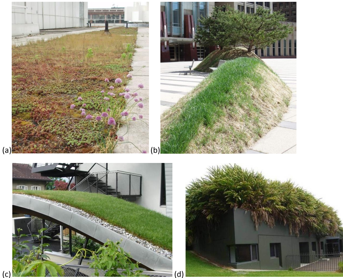
Figure 9. Examples of (a) simple or (b) difficult living roofs to maintain, (c) no mower access, no balustrade and loose gravels can be thrown by a lawn mower or weed whacker (safety), (d) overgrown with difficult access and inability to see the building edge.
