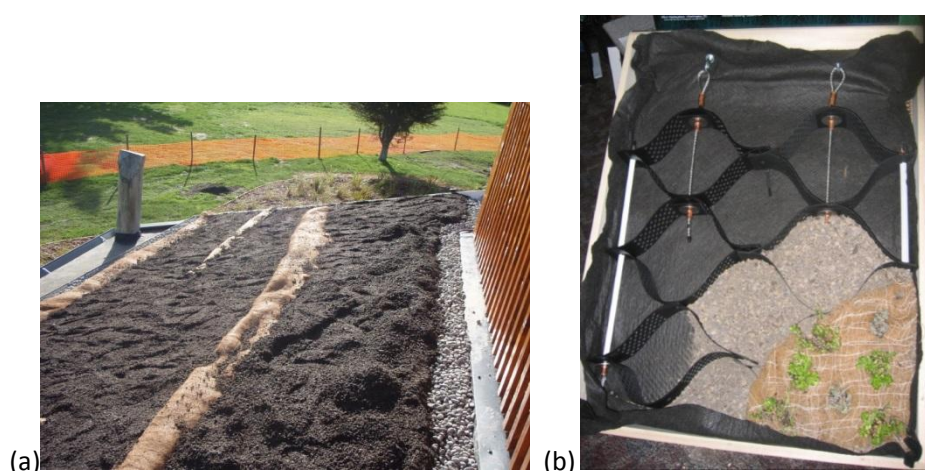
Figure 6. (a) Coconut coir slope breaks on the Auckland Botanic Gardens 15° pitch living roof; (b) commercially-sourced flexible synthetic matrix to prevent substrate migration.
