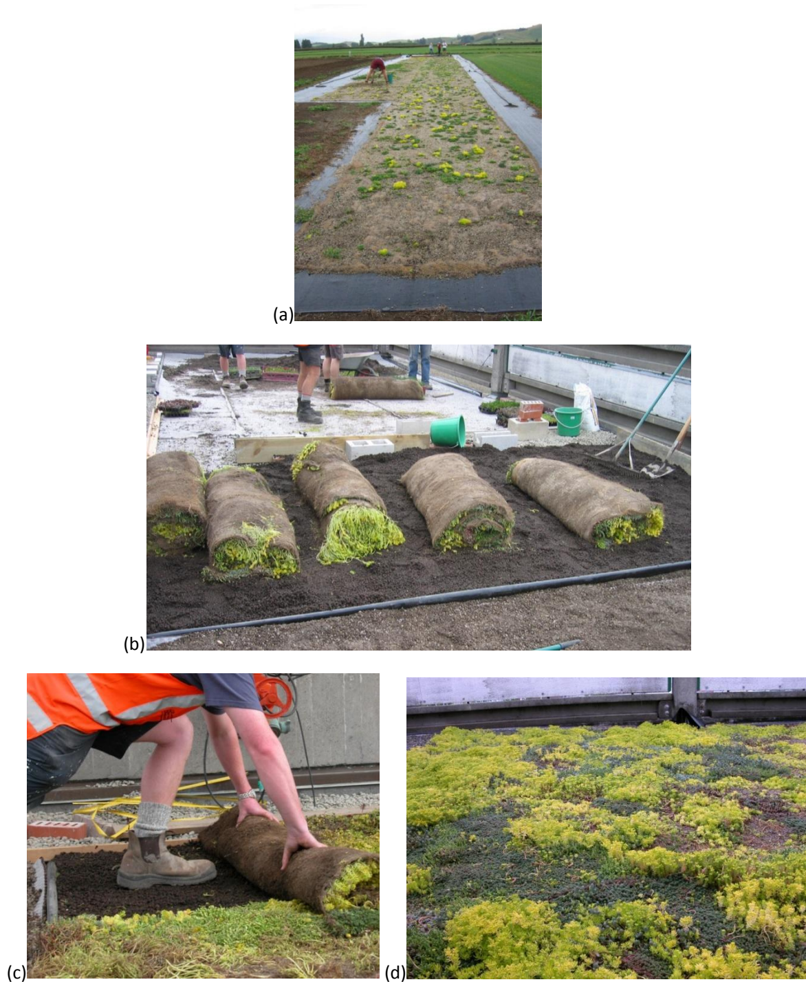
Figure 27. Pre-grown mat: (a) establishment; (b) arrival on-site (c) installation; (d) instantaneous effect
