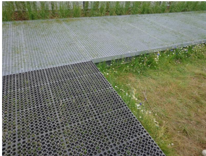
Figure 16. Rigid drainage boards allow foot traffic without damage to vegetation or compromising drainage.
