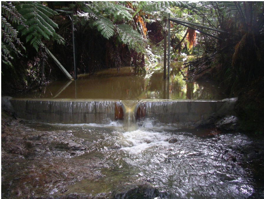
Figure 1.2: Photograph of the v-notch weir at Okura - Weiti Stream flow recording station.
