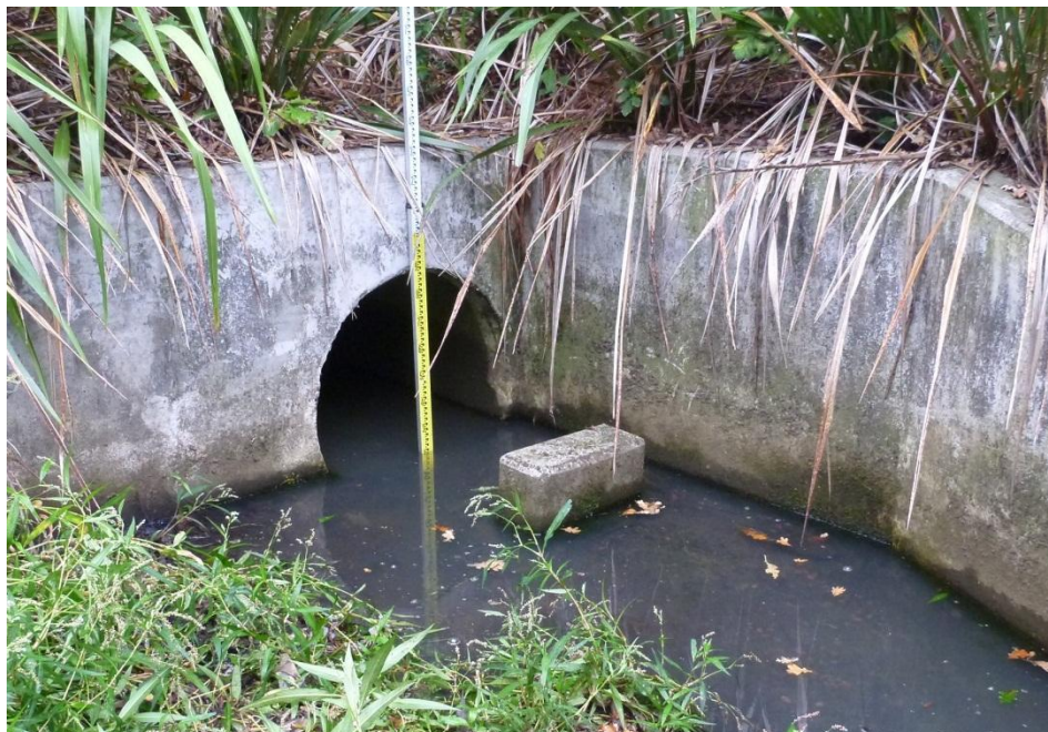
Figure 23: Concrete Aprons with Baffle Blocks Embedded for Energy Dissipation
