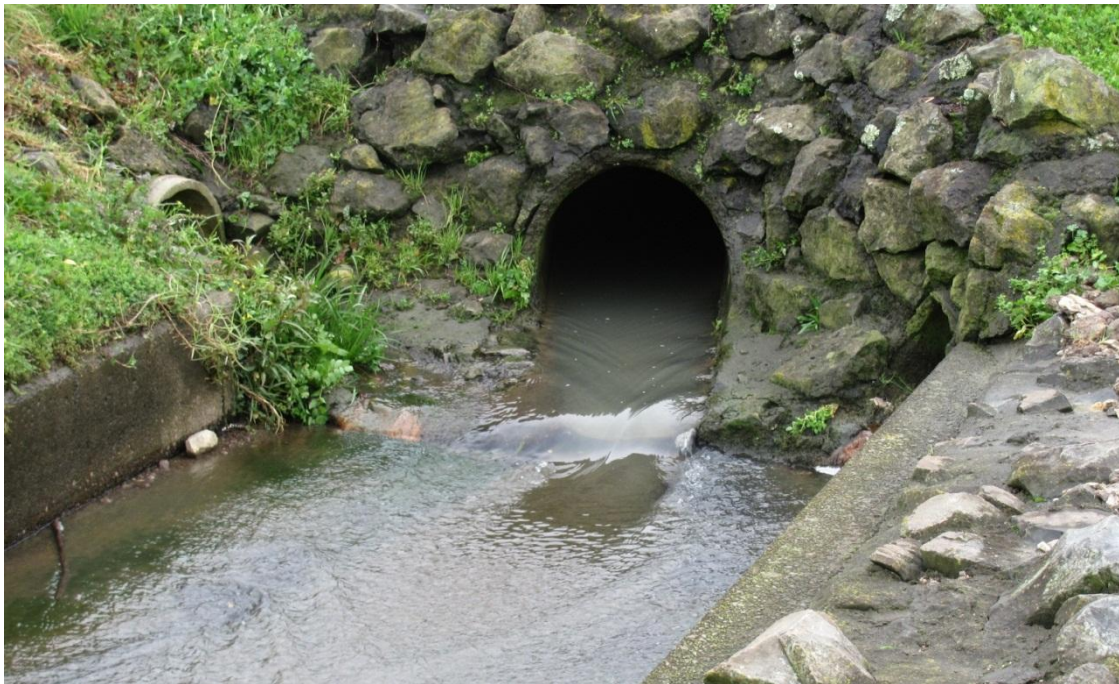
Figure 37: Grouted Rock Headwall
