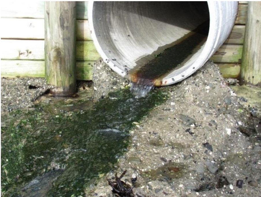
Figure 35: Culvert Apron with Cement, Sand and Shell Natural Finish
