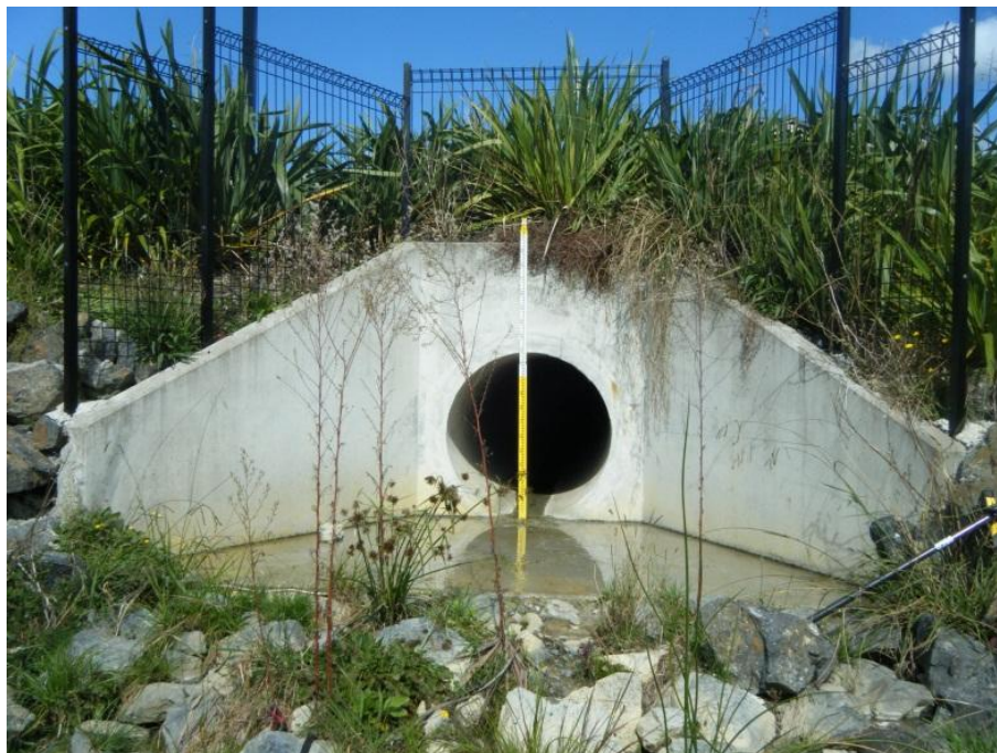
Figure 20: Standard Wing-wall Outlet with Apron, Fencing, Planting and Downstream Riprap
