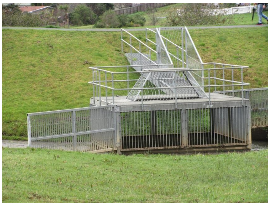
Figure 46: Large Inlet Structure with Maintenance Access and Numerous Grilles
