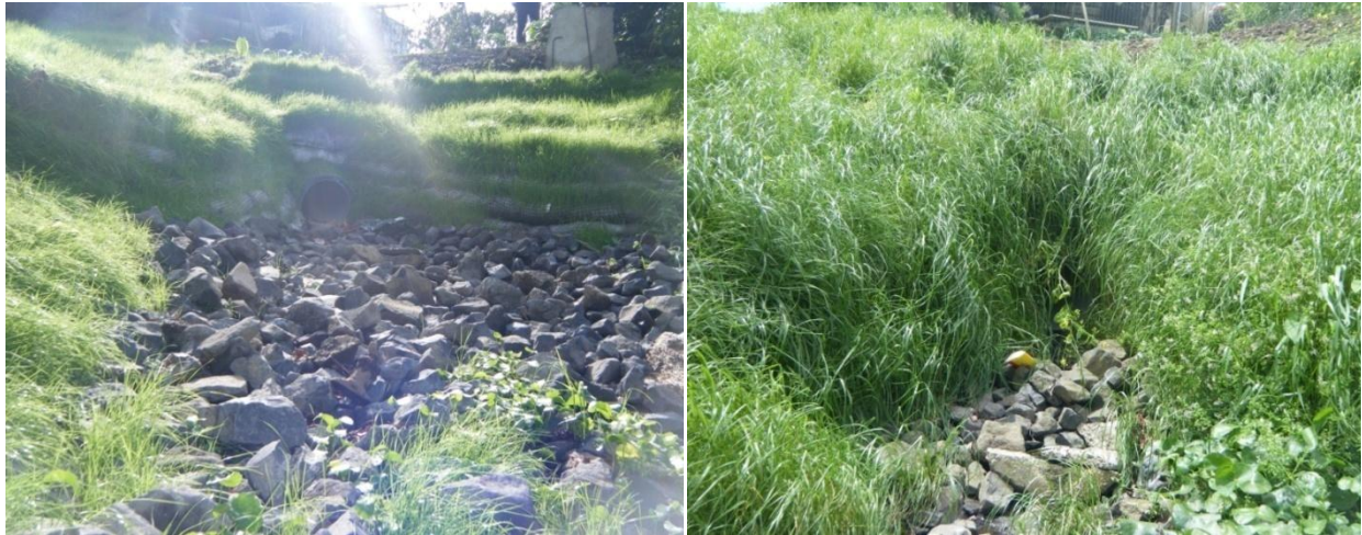
Figure 38: Outfall with Riprap and "Living Wall" Confined Earth Retaining Structure
