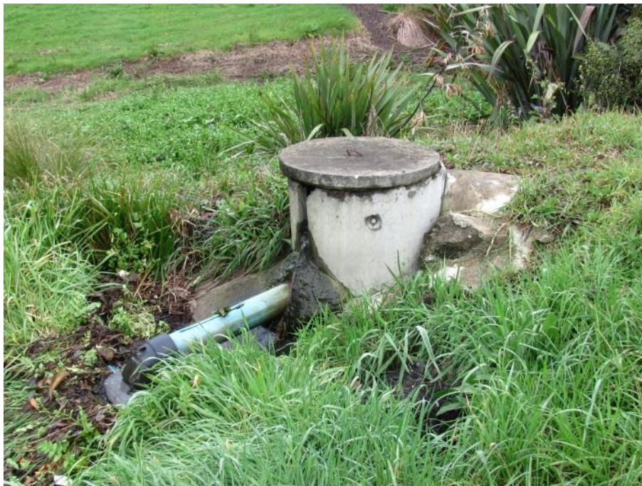
Figure 1: Poorly Designed, Poorly Constructed Rain Garden Inlet in a Public Reserve
