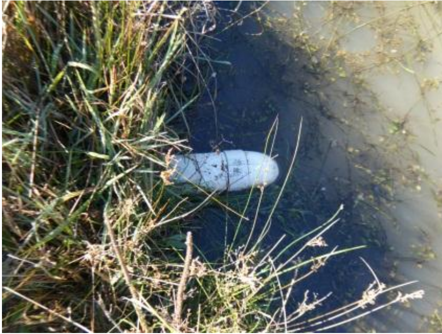
Figure 41: Downturned Bend on Simple Outlet
