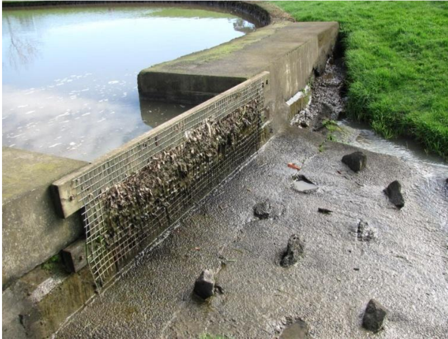
Figure 43: Poorly Built Retrofitted Debris Grille
