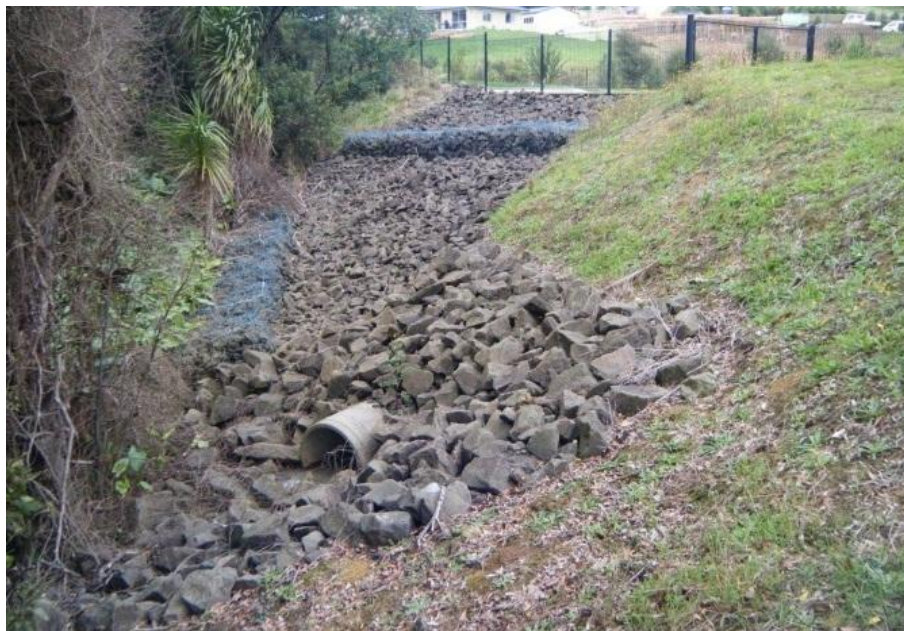
Figure 16: Riprap with Check Dam at Pond Spillway
