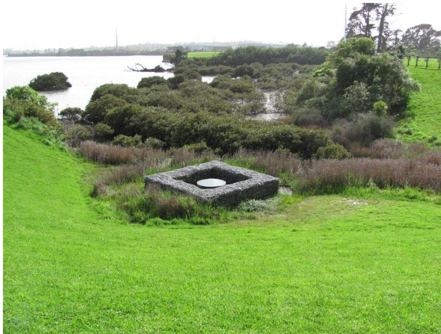
Figure 40: Gabion Basket Outlet
