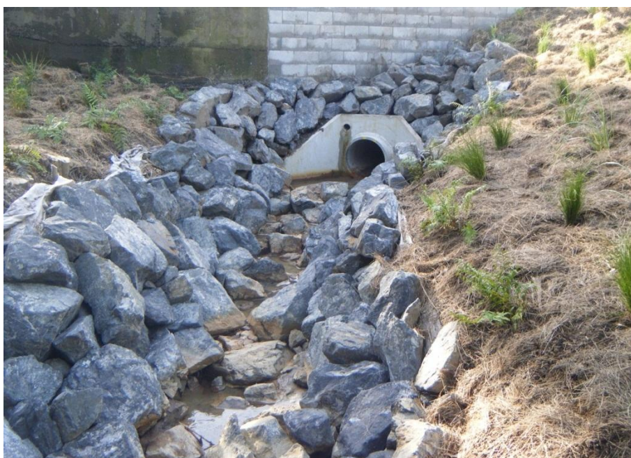
Figure 17: Riprap Protection and Dissipation and Pipe Outfall
