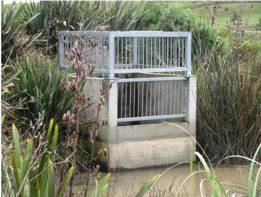
Figure 12: Outlet with Weir and High Level Intake
