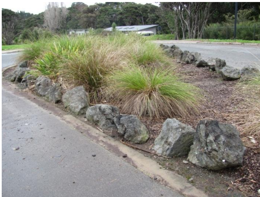
Figure 4: Boulders Distribute Inlet Flow
