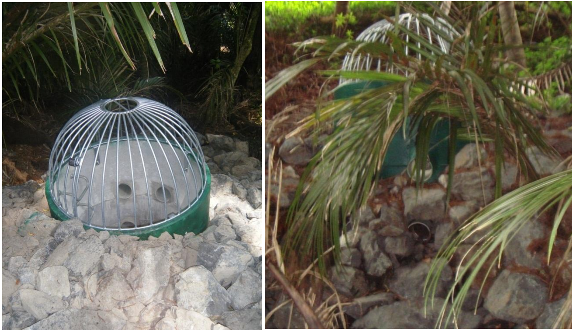
Figure 27: Bubble up Pit in Bush Gully Looking Downstream (left) and Upstream (right)
