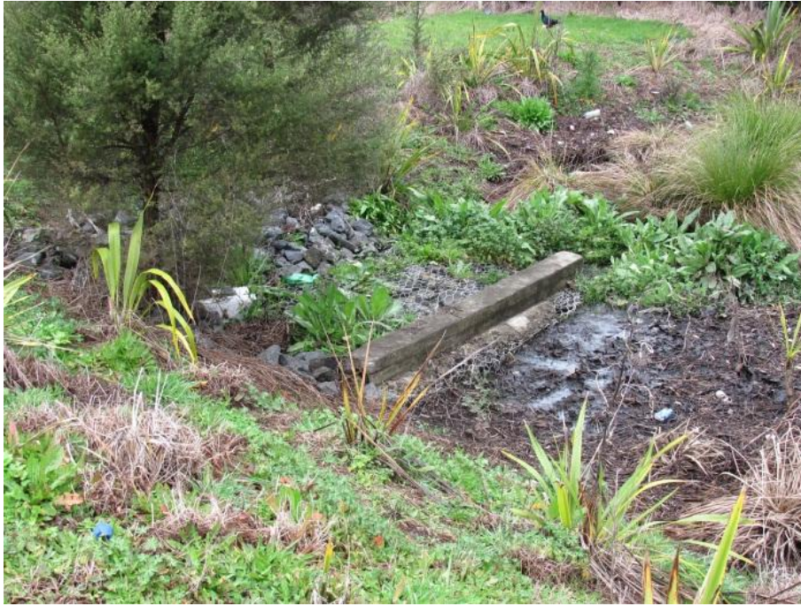
Figure 8: Poorly Designed and Constructed Level Spreader
