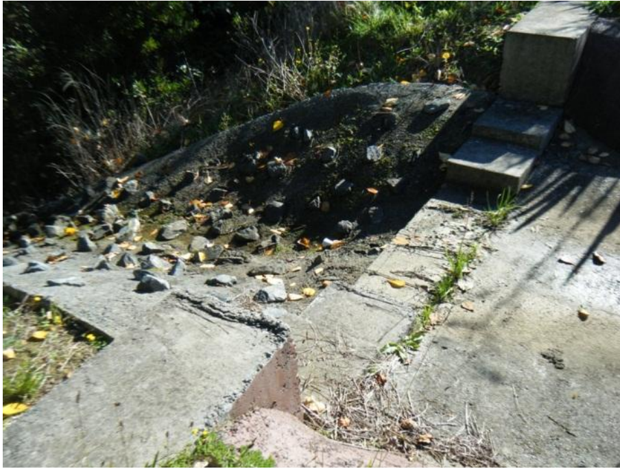
Figure 34: Poor Finish on Concrete Weir
