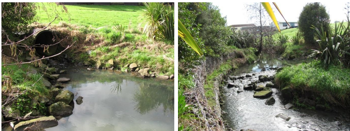
Figure 28: Outfall with Channel Rock Protection and Gabions to Protect Opposite Bank
