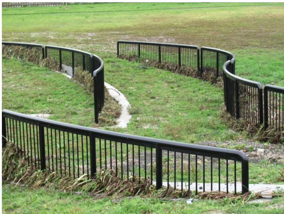
Figure 45: Effective Debris Fencing Upstream of Critical Inlet
