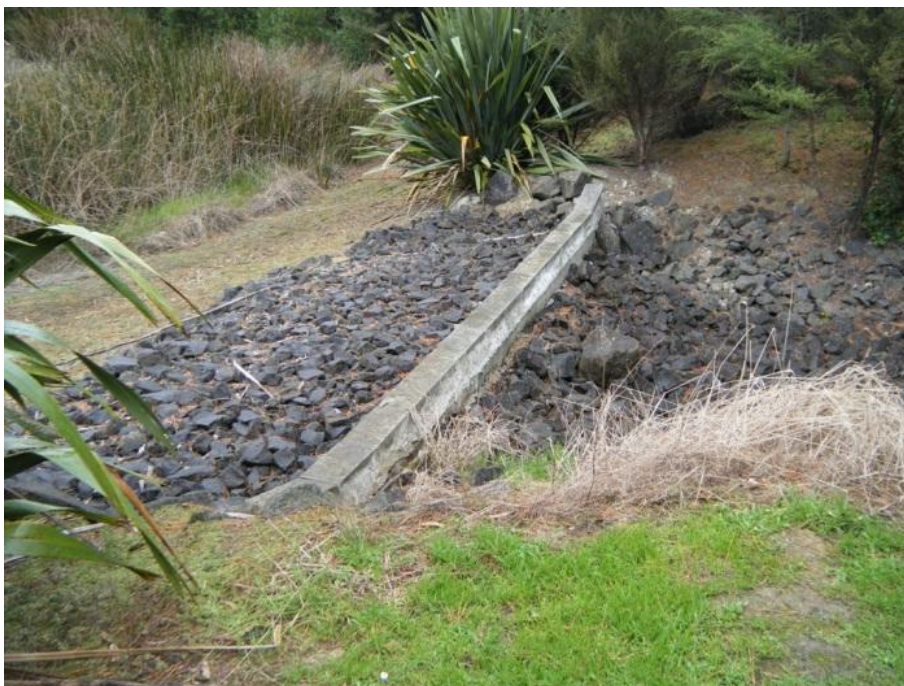
Figure 9: Well Designed and Constructed Concrete Beam Level Spreader
