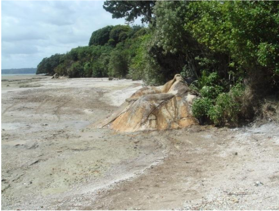
Figure 36: Outfall Energy Dissipation with Natural Finish
