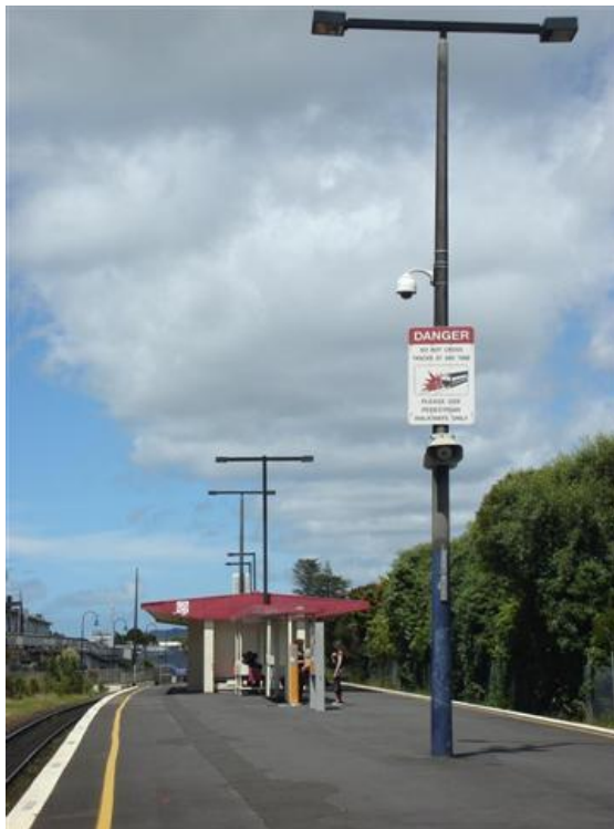
(Photo: Ken McLeod, Auckland Transport)
