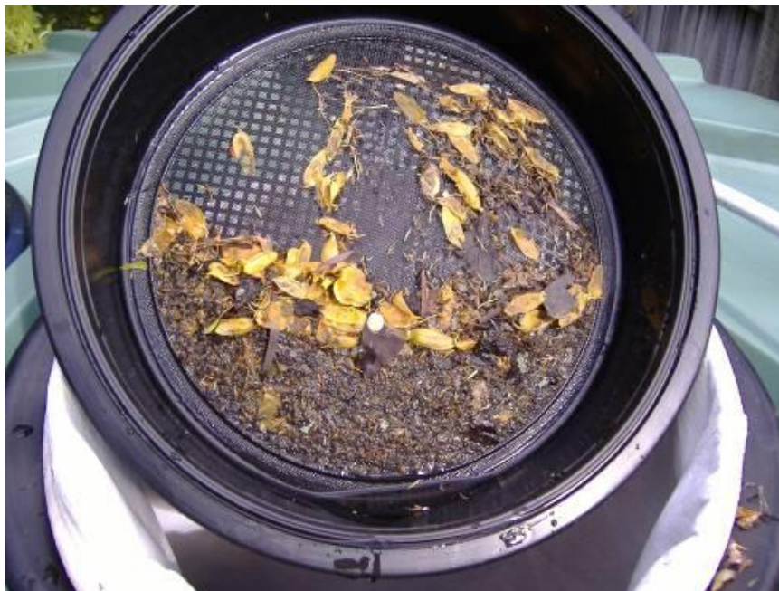
Figure 86 Rain tank filter showing leaf litter and organic debris.
