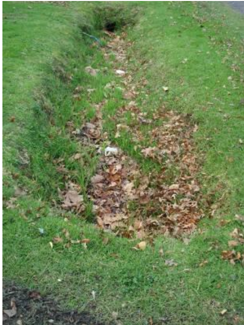
Figure 35 Road side urban swales.
