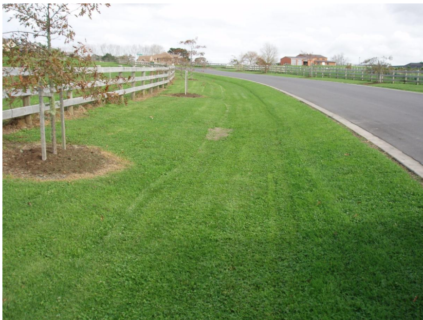
Figure 36 Goodlands Estate greenfield development roadside swale.
