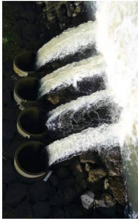
Fig. 60 Total barrier - swimming and climbing species unable to pass
