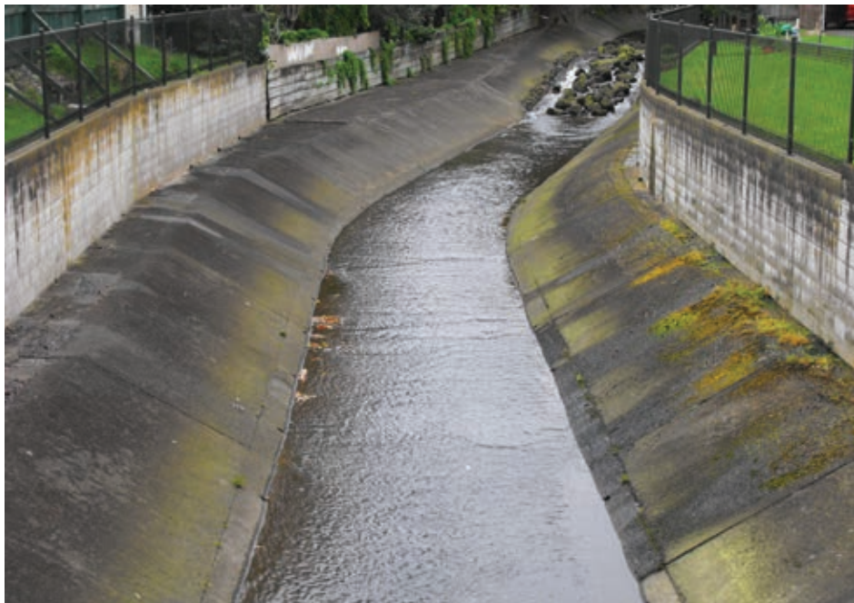
Fig. 41 Bank and bed lined with impermeable artificial lining
