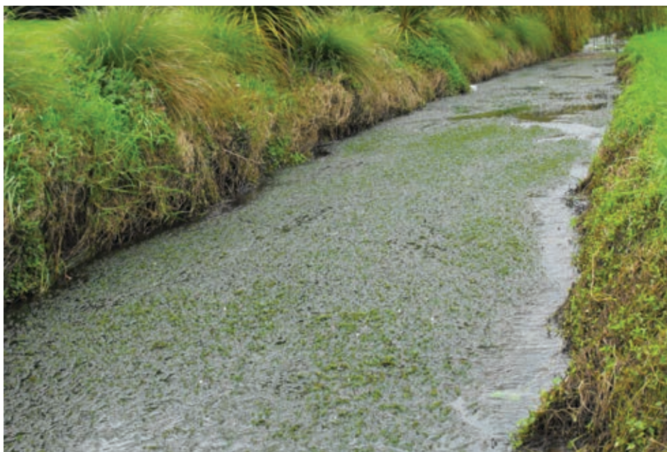
Fig. 33 Channel affected by increase in roughness elements
