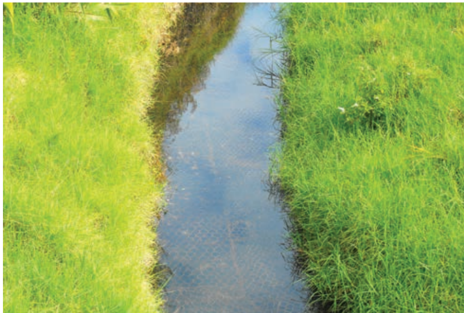
Fig. 38 Bed lined with permeable artificial lining
