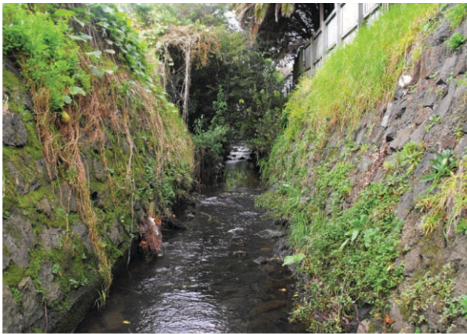
Fig. 81 Riparian root zone connection limited by channel lining
