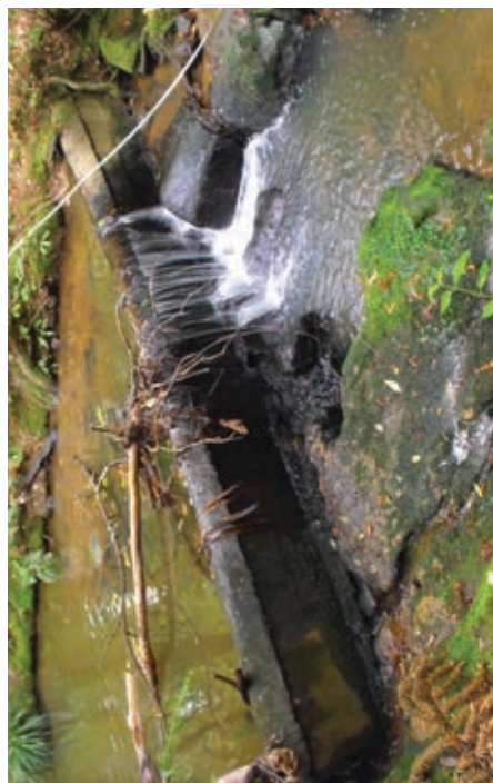
Fig. 59 Partial barrier - swimming species unable to pass
