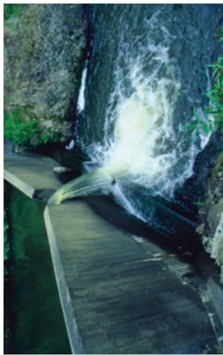
Fig. 61 Total barrier - swimming and climbing species unable to pass
