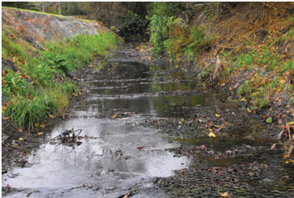
Fig. 40 Bank and bed lined with permeable artificial lining
