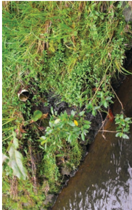
Fig. 26 Single piped inflow, less than 20cm in diameter
