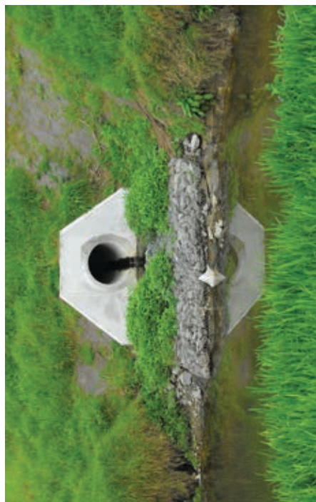
Fig. 29 Single piped inflow, greater than 20cm in diameter
