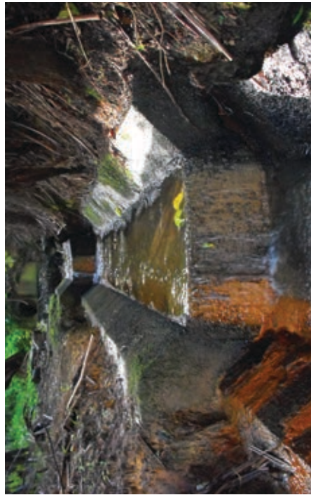
Fig. 58 Partial barrier - swimming species unable to pass
