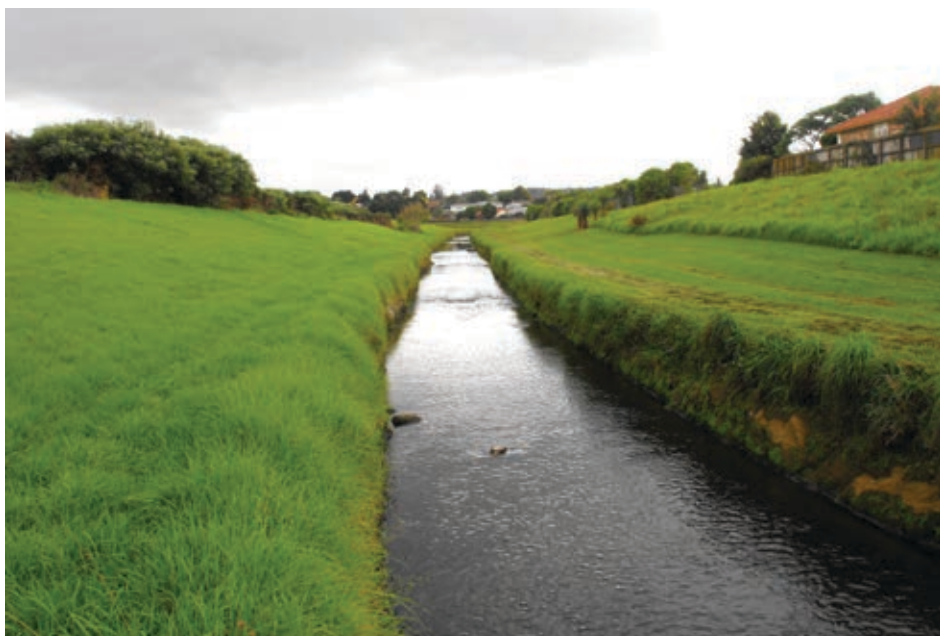
Fig. 35 Channel straightened and deepened
