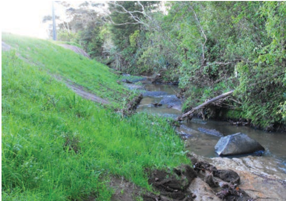
Fig. 31 Upper bank widened to increase capacity
