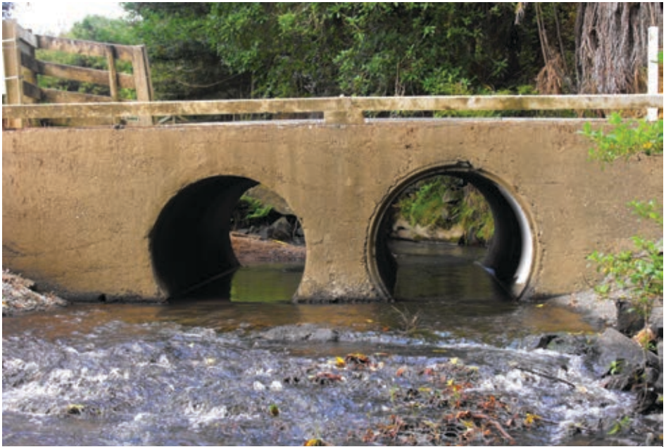
Fig. 80 Riparian root zone connection limited by culvert
