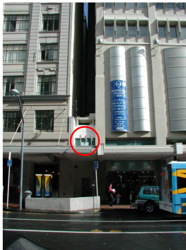
Figure 7.3 Photo of Queen Street monitoring site with sampling inlets circled in red
