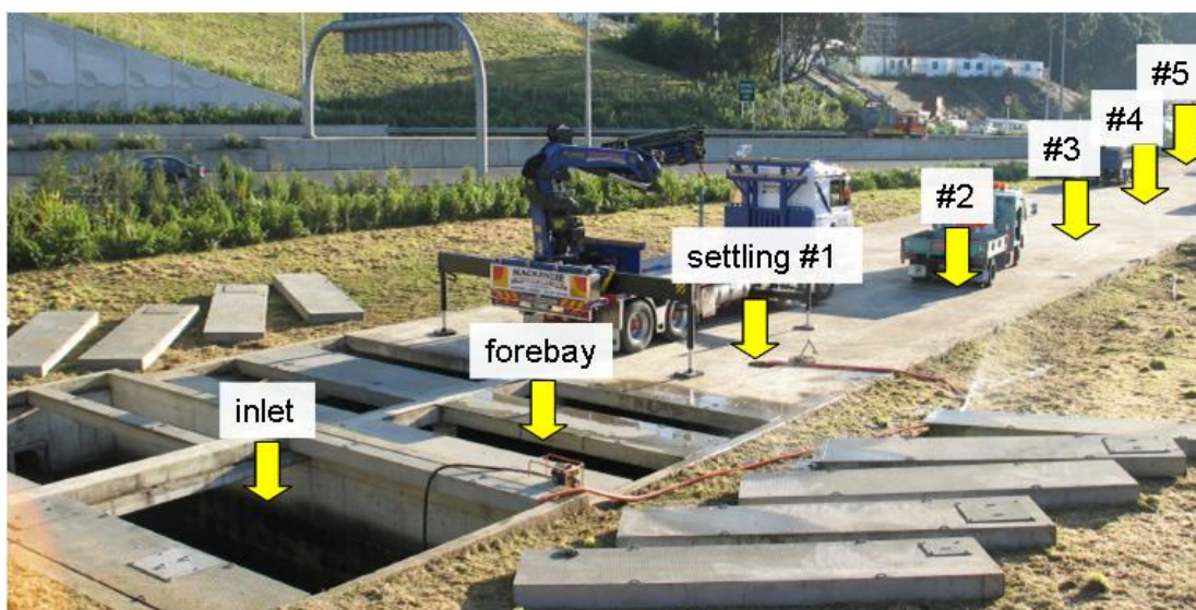
Figure 1 Sample locations within the retention tank.
